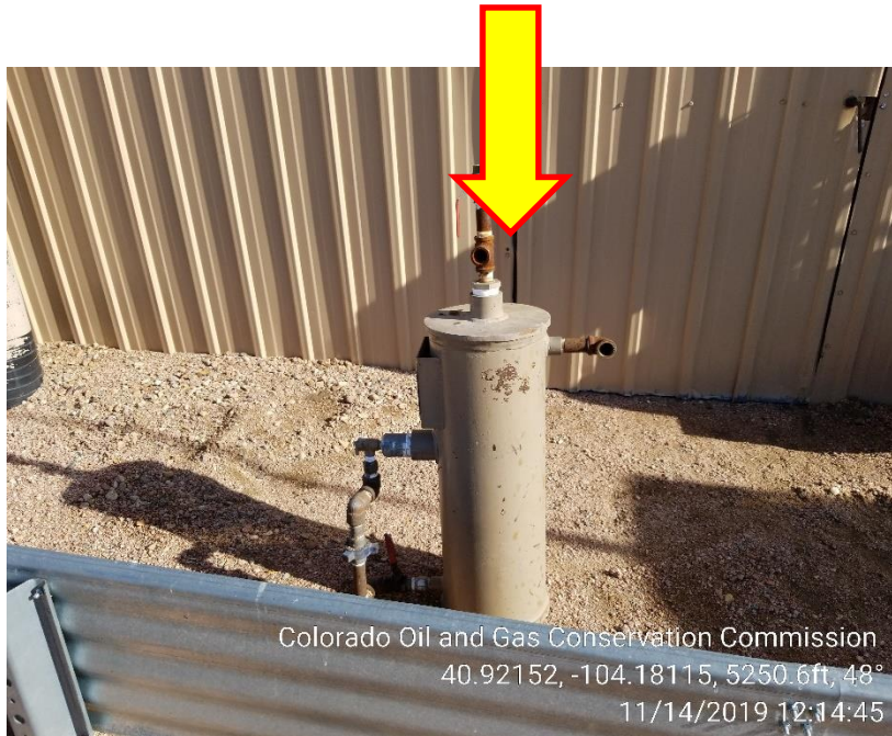
Photo 5 – Unused Supply/Volume Vessel
