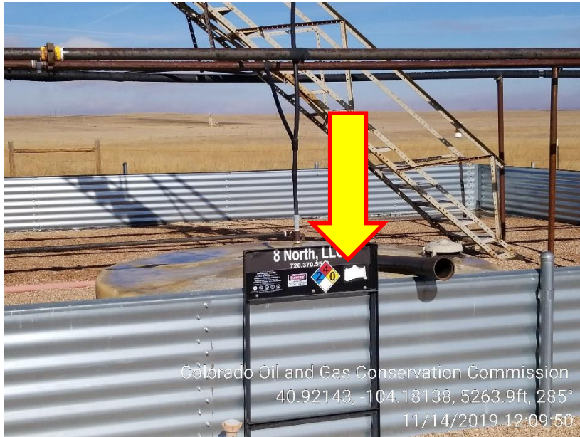
Photo 3 – Fiberglass Vault – Capacity has faded no longer legible
