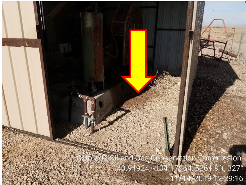
Photo 3 – Stained Soil at Gas Engine
