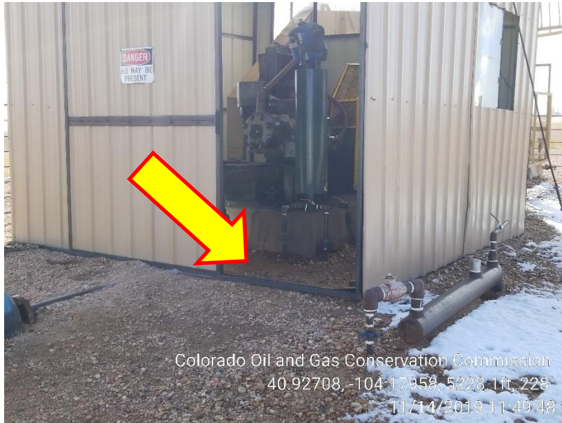
Photo 3 – Stained Soil at Gas Engine
