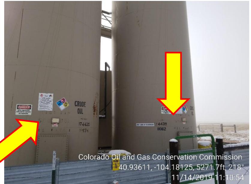
Photo 2 – Capacity Labels have faded no longer legible
