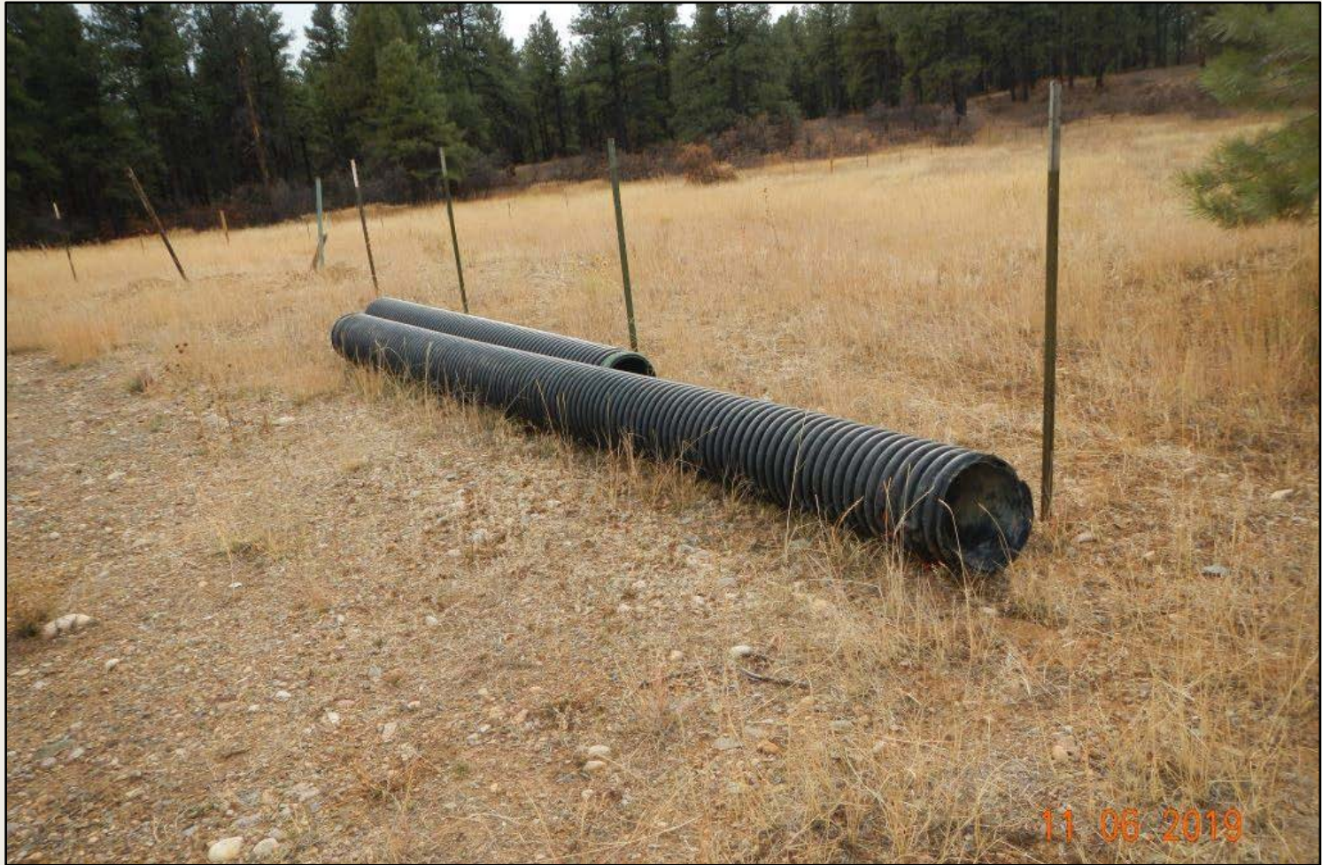
Photo 3. View of black pipes within the southwestern project area that need to be removed.
