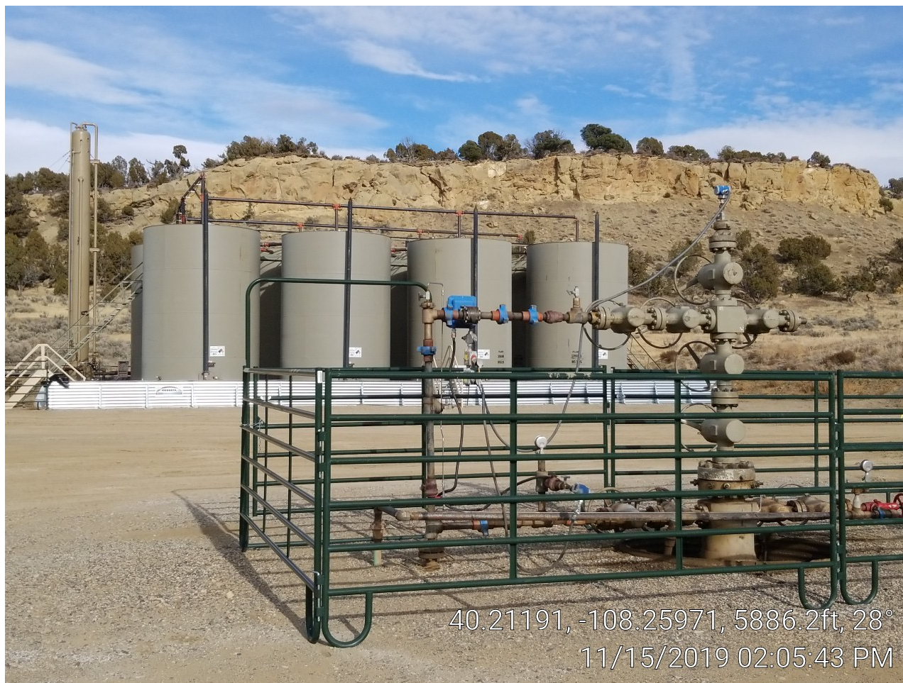
Photo 2. Tank battery & well head.
