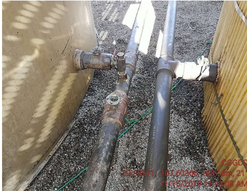
Stained gravel and paraffin on piping
