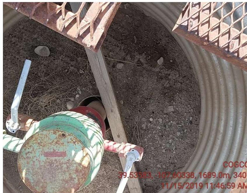
Wildlife escape board not positioned
