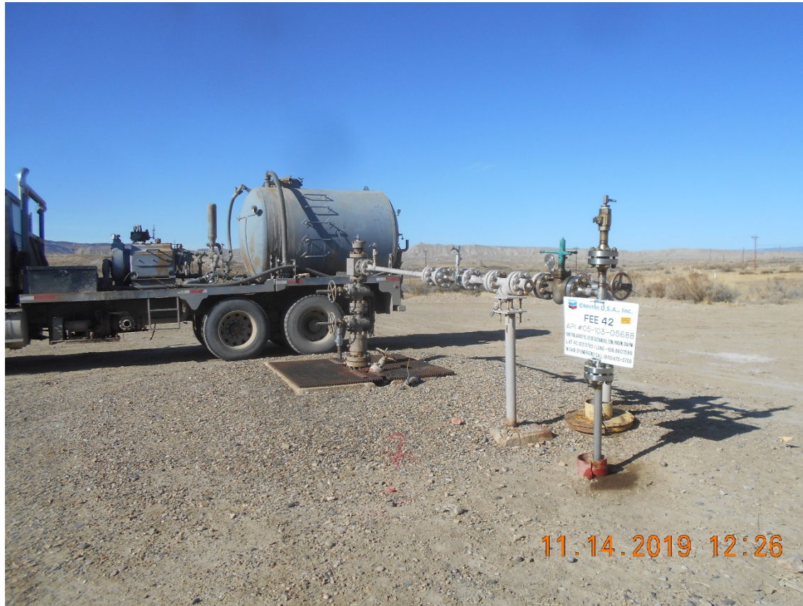
Injection Wellhead.
