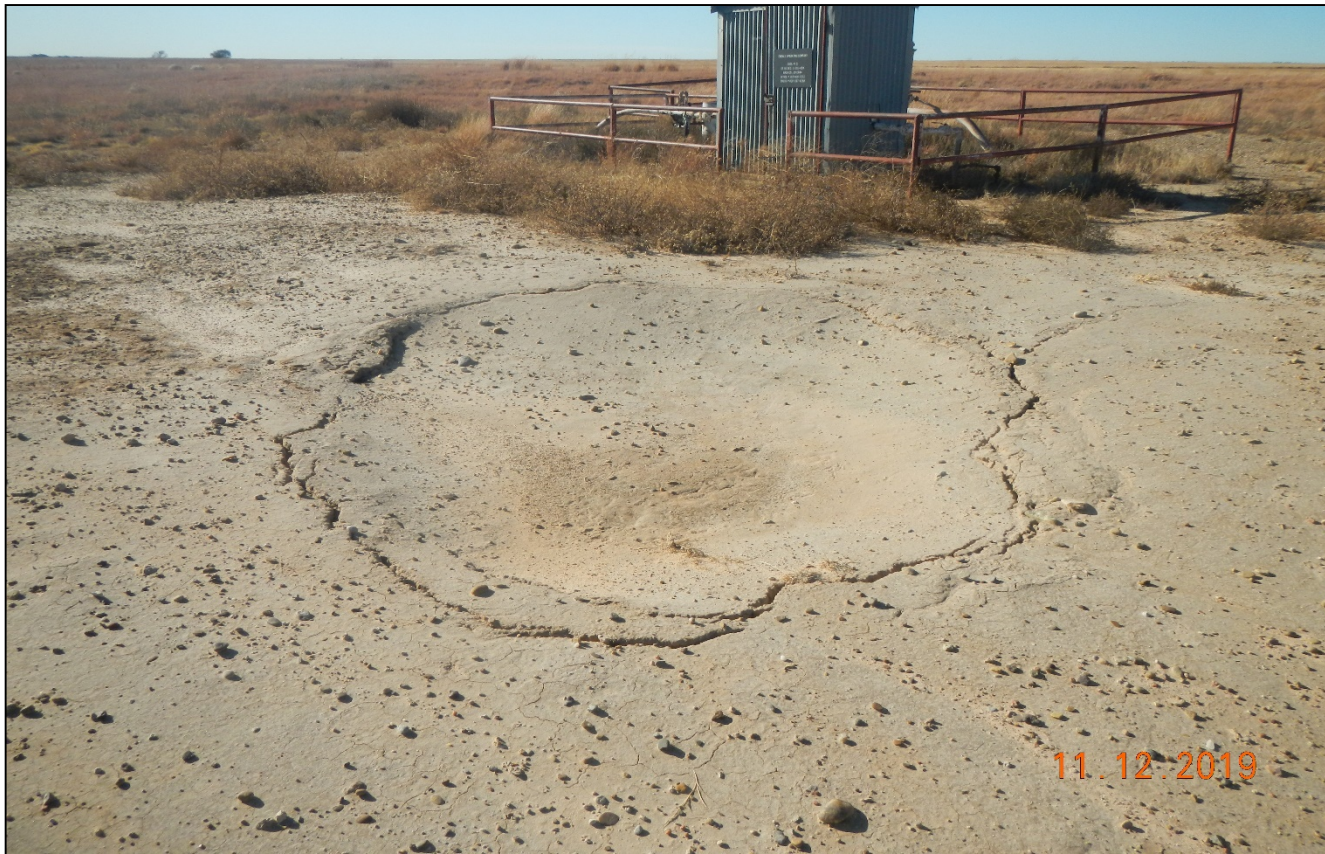
Photo 4. There is an area of subsidence near at the location approximately 8x8 ft.
