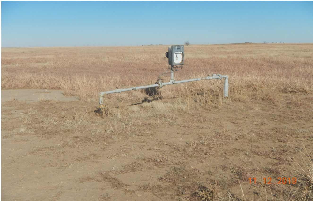
Photo 3. There is a meter pipe riser that remains at the location. All equipment must be removed.
