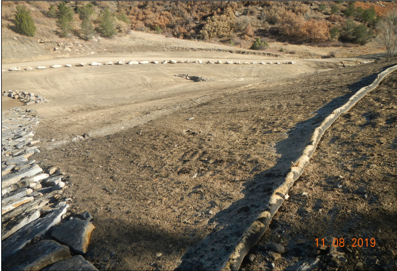
Photo 3. Erosion controls are installed along the slope.
