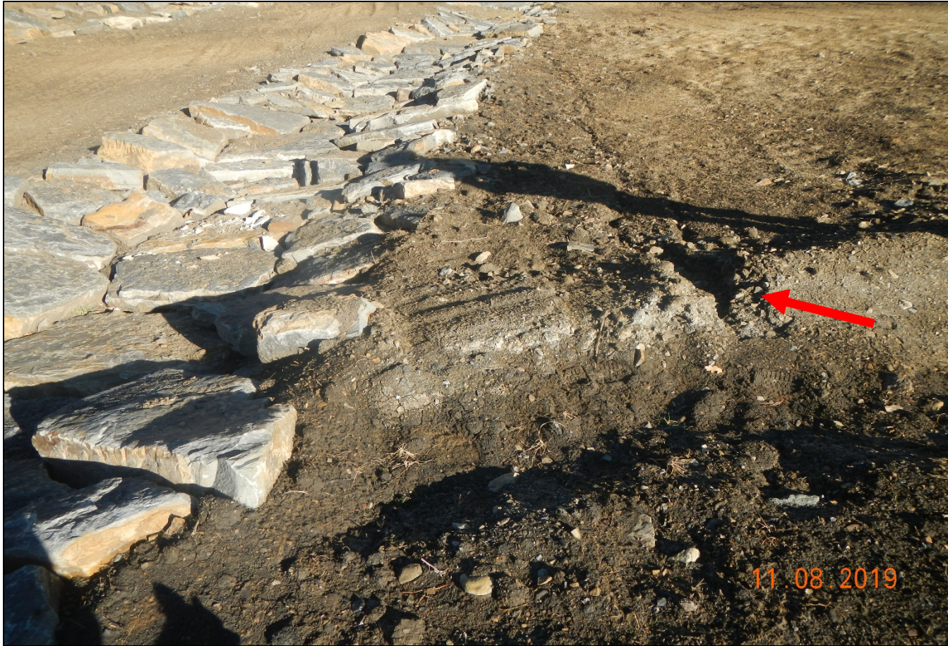
Photo 4. Stormwater has begun to degrade the berm. Stormwater should be diverted toward the rock rip rap structure and berm needs to be repaired.
