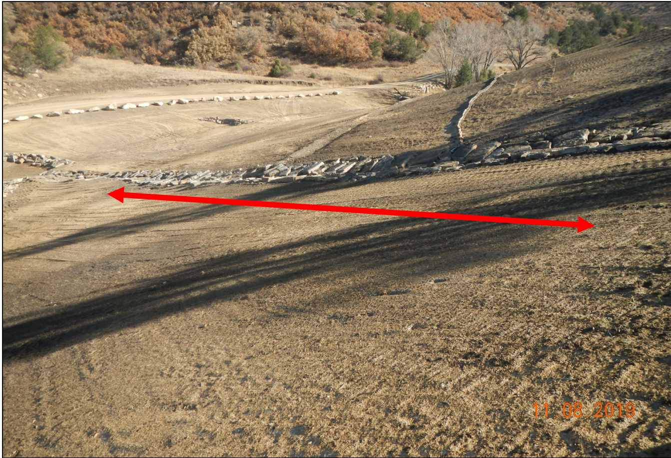
Photo 5. Facing northeast along the slope of the reclaimed location. This slope may need additional BMP's (Wattles) to slow the stormwater runoff.
