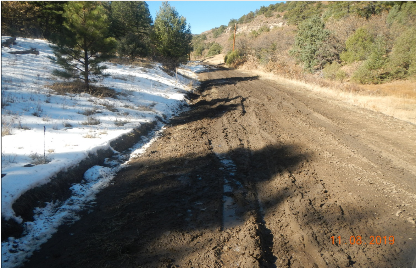
Photo 2. There are vehicle ruts and road damage along the main road to the location. This area is very slick and is a safety issue. The road requires gravel in this area.
