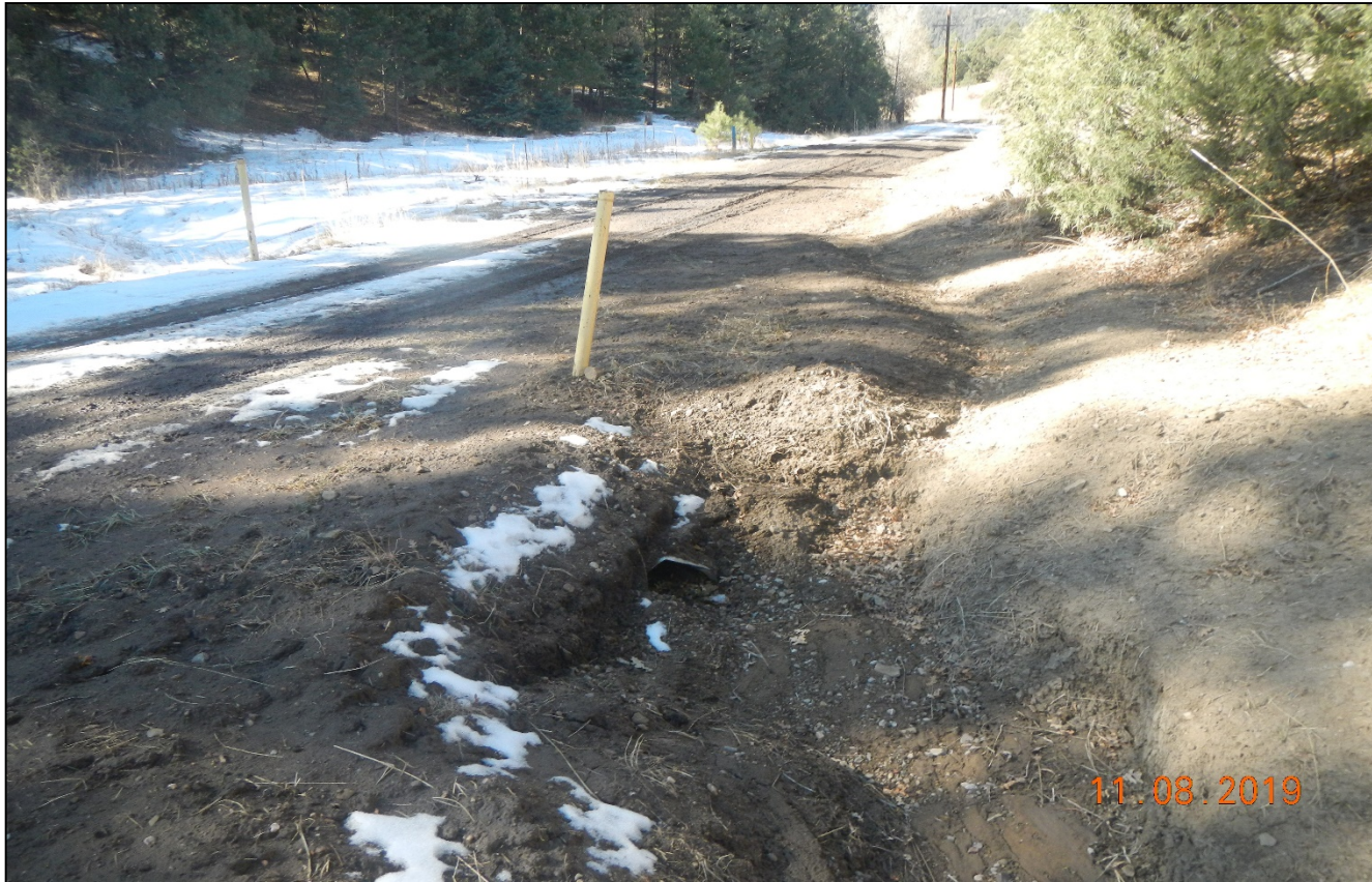
Photo 3. Sediment is beginning to accumulate in the culvert outlet at the stream crossing.
