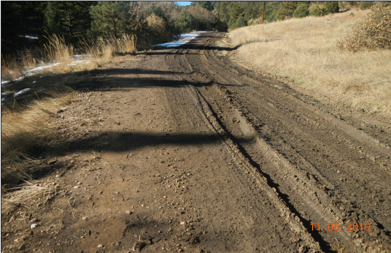
Photo 1. There are vehicle ruts and road damage along the main road to the location. This area is very slick and is a safety issue. The road requires gravel in this area.
