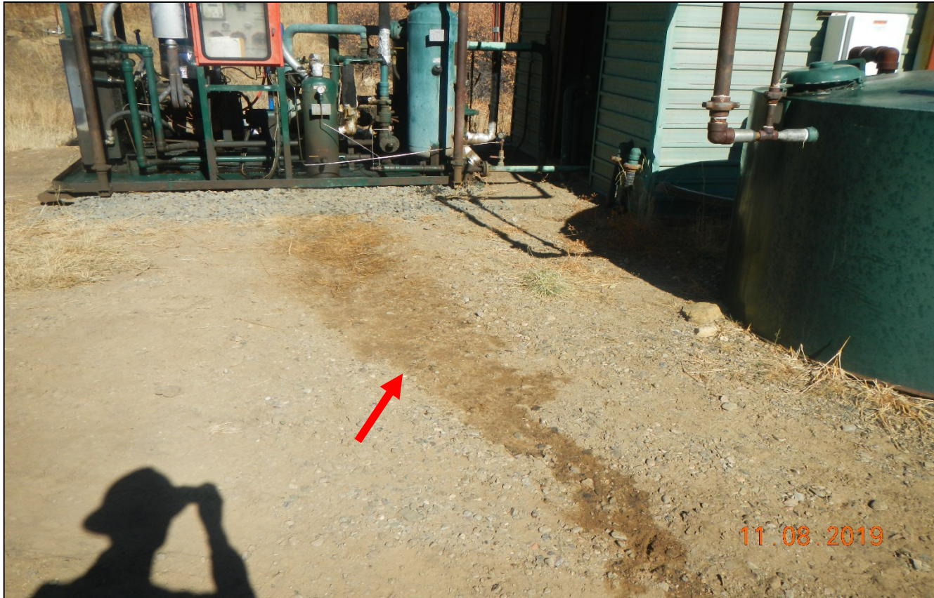
Photo 5. There is an area of oil stain soil near the engine skid that needs to be cleaned up.
