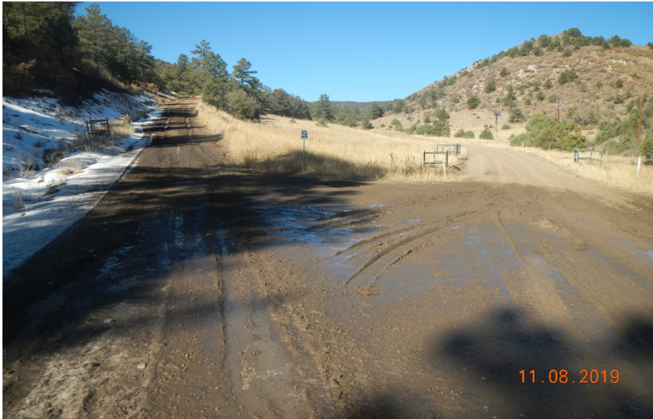
Photo 1. Stormwater is not properly diverted off the road at this point. This issues is causing vehicle ruts and road damage.
