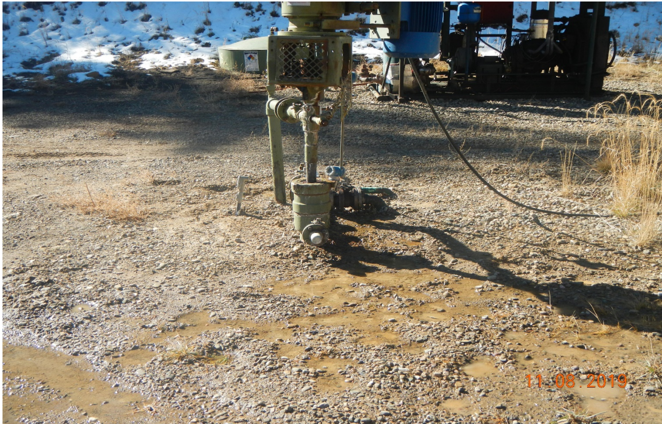
Photo 2. The water leak at the wellhead has not been repaired.
