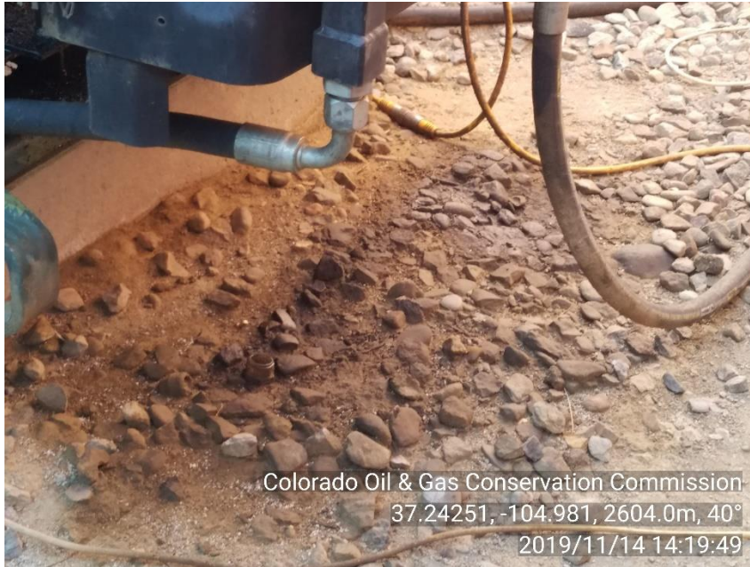
PHOTO 3: AREA OF IMPACTED SOIL NEAR PRIME MOVER (ENGINE SKID). Remove and dispose impacted material in approved manner, service and maintain equipment and self inspect to prevent recurrence of conditions per 1002.f(2) and 907. CA DATE 12-14-19.
