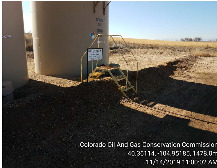
Crude oil tank berm
