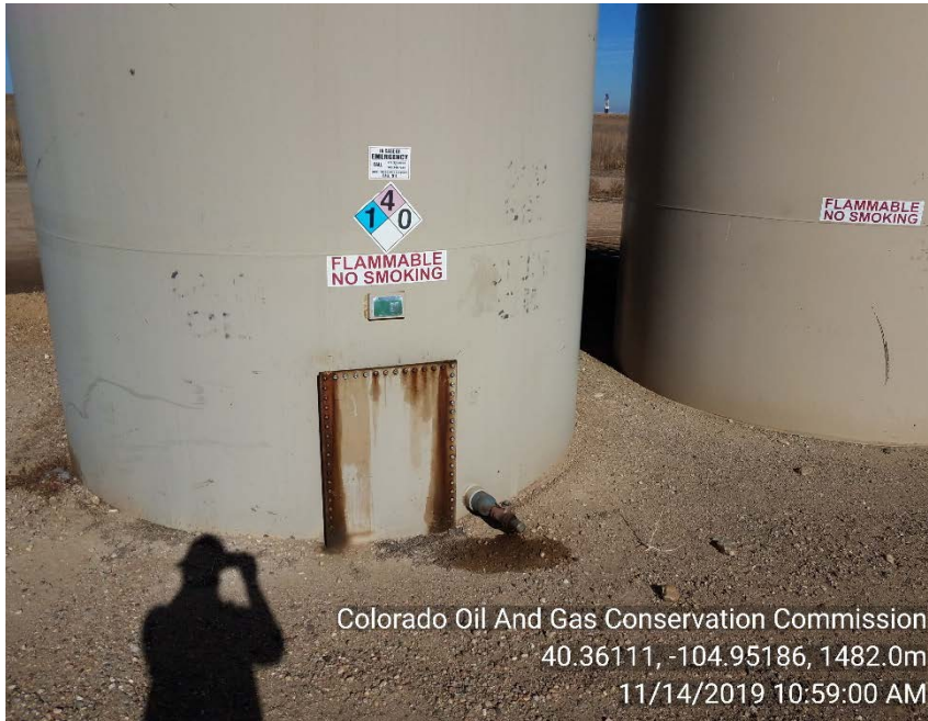
West crude oil tank leaks and stained soil
