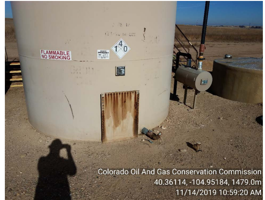
East crude oil tank leak
