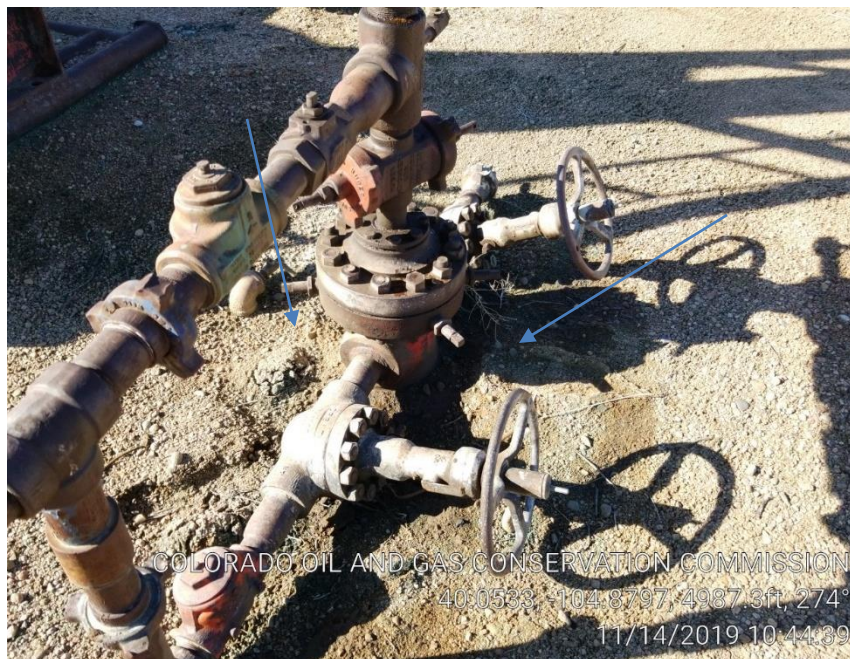
Pic 1 stained soil/mechanical issue on wellhead
