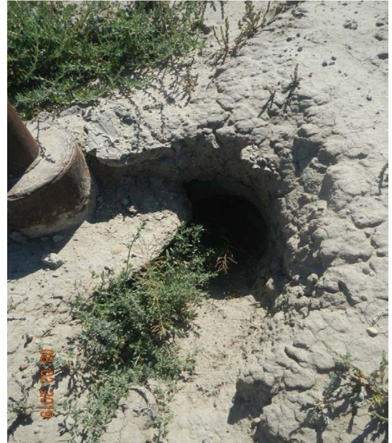
Photo#4: View of subsidence at base of Marker.
