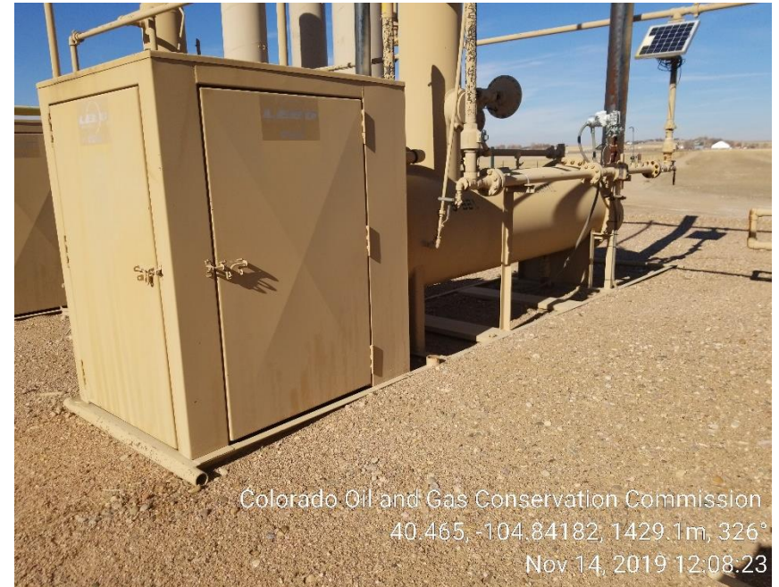
Photo 32: Separator not anchored
