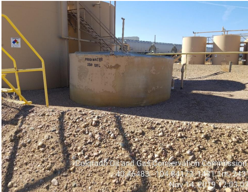
Photo 27: No NFPA placard on tank/Tank not anchored
