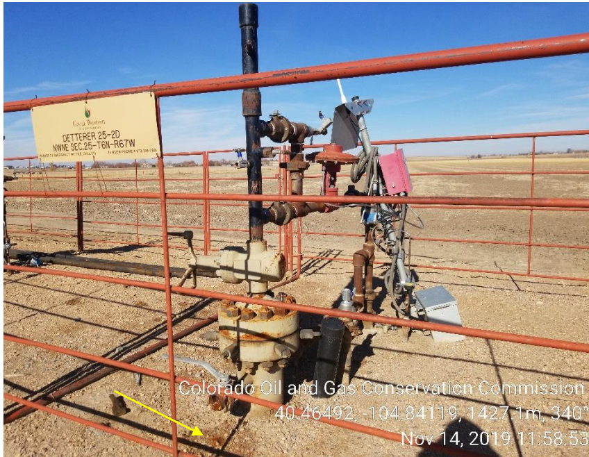
Photo 13: Wellhead/stained soil
