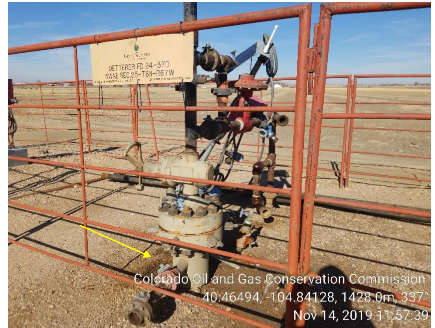
Photo 6: Wellhead/ stained soil
