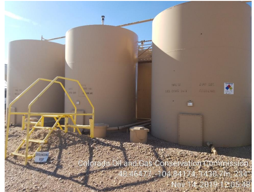
Photo 28: Tanks not anchored
