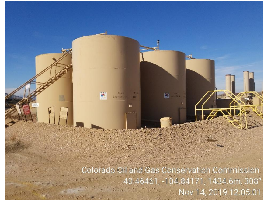
Photo 26: Tank Battery/inadequate berm
