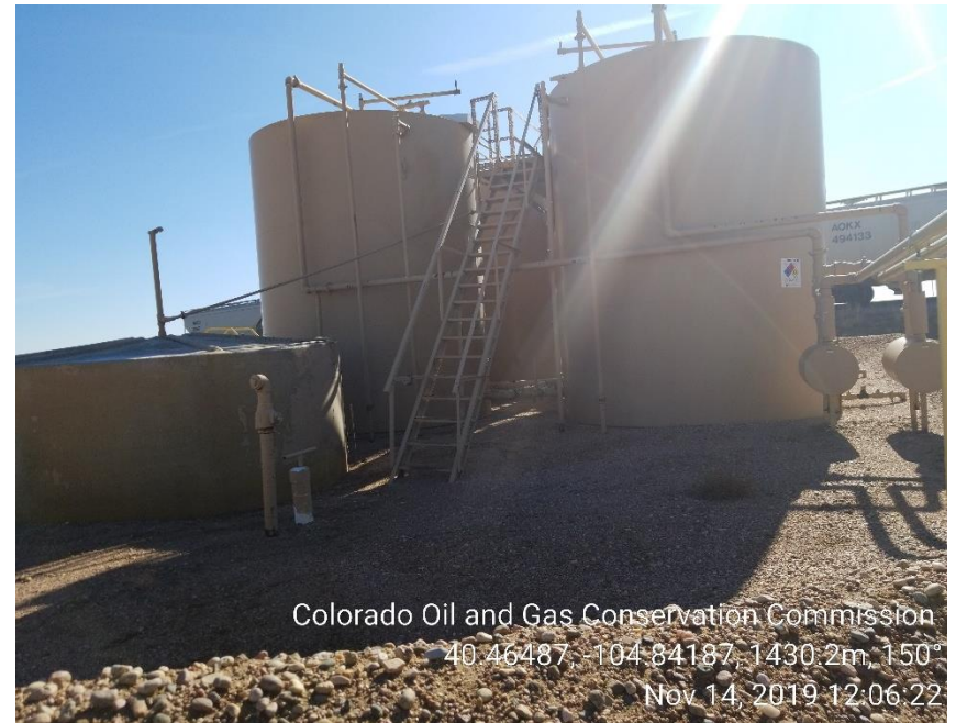
Photo 30: Tanks not anchored
