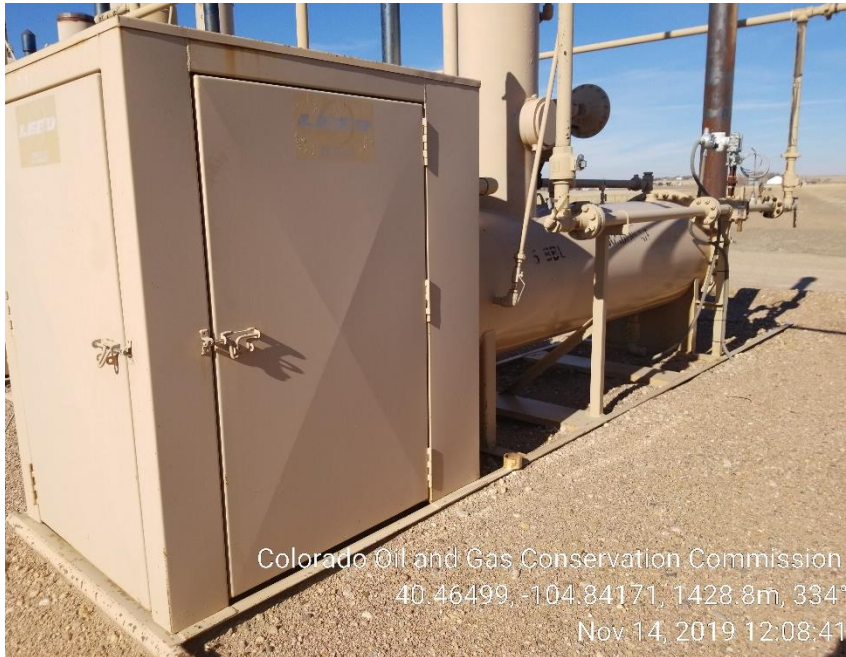
Photo 35: Separator not anchored
