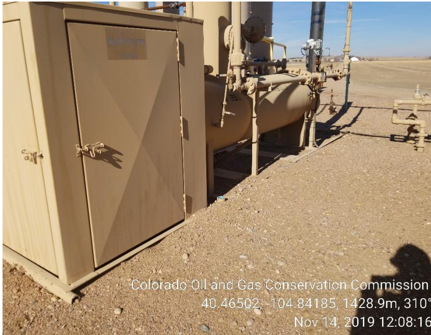
Photo 31: Separator not anchored
