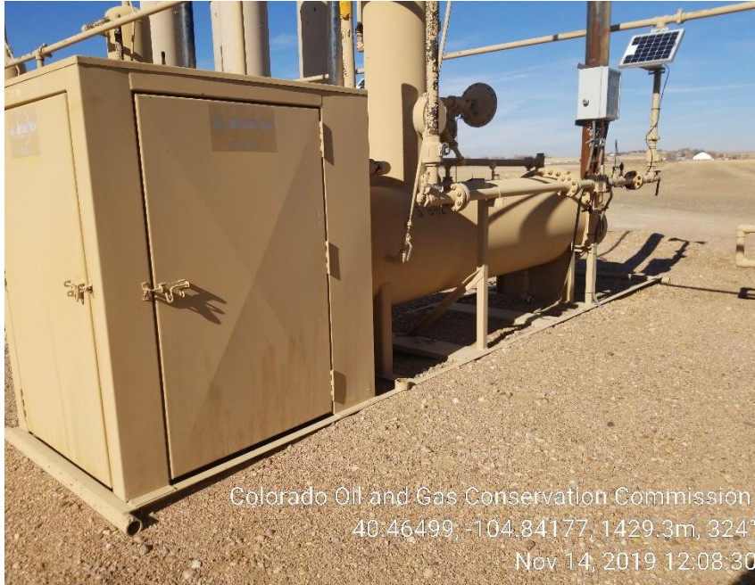
Photo 33: Separator not anchored
