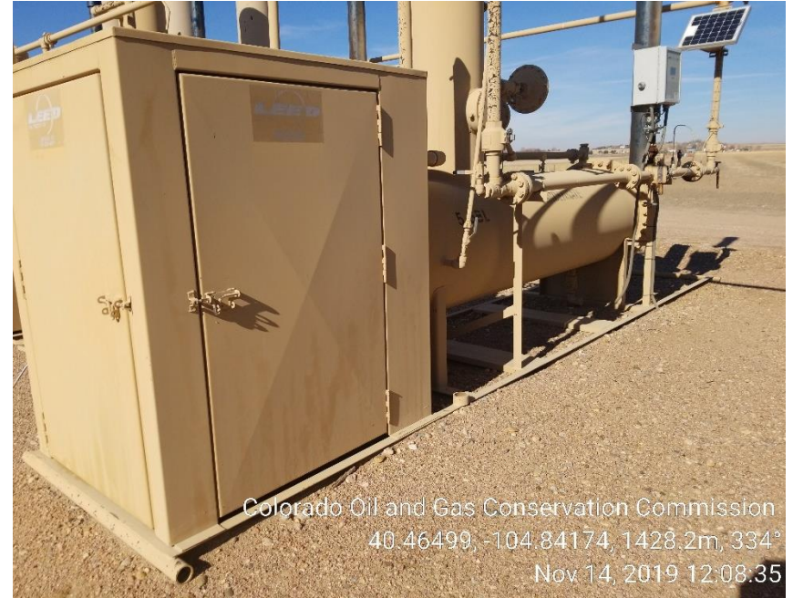
Photo 34: Separator not anchored
