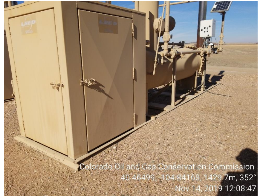
Photo 36: Separator not anchored
