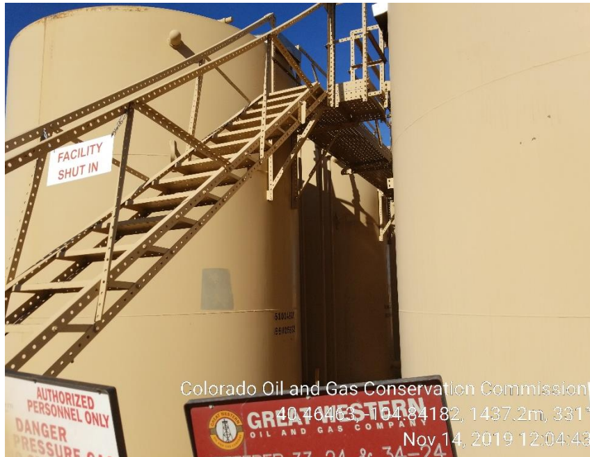
Photo 29: Tanks not anchored
