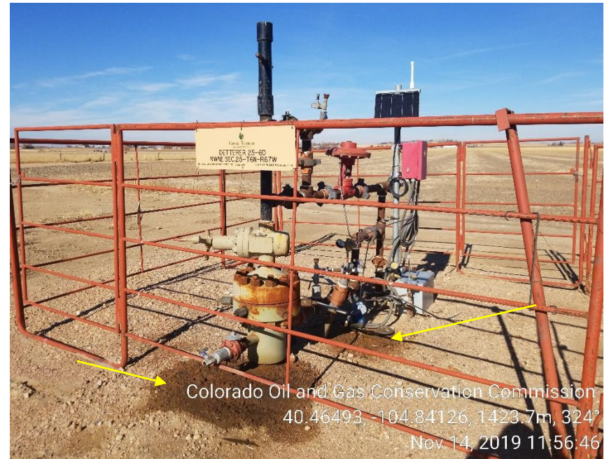
Photo 2: Wellhead/stained soil
