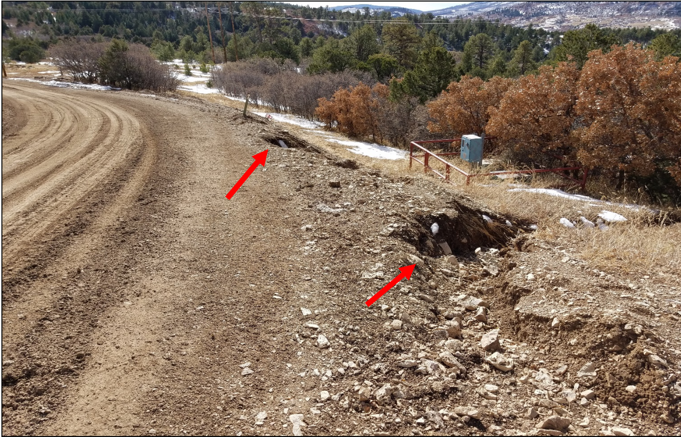
Photo 1. There is erosion occurring along the access road to the location. Stormwater is directed off the road at the point creating an erosion channel. Lat/Long:37.70081,-105.20980.
