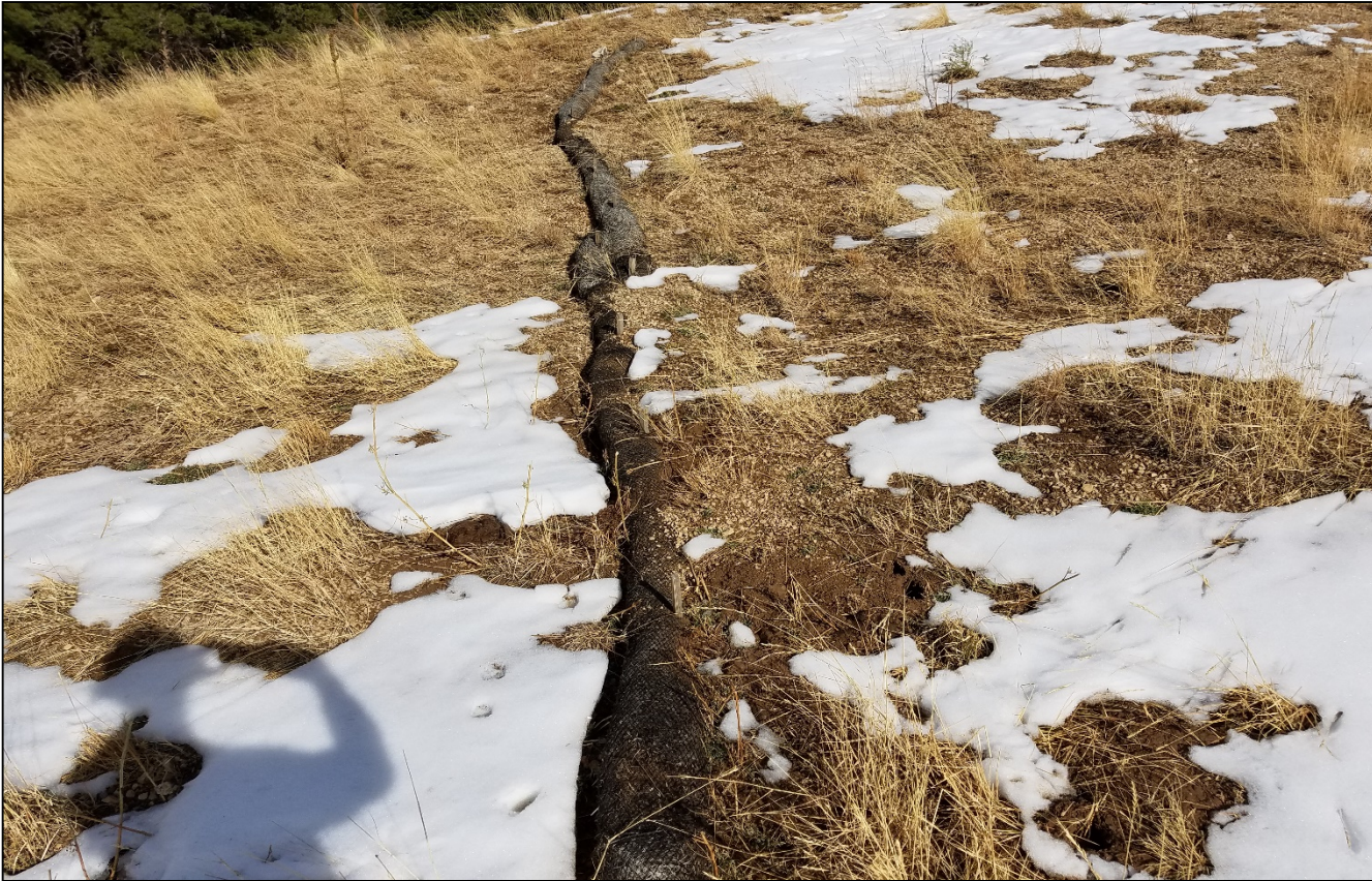
Photo 8. This wattle has filled in with sediment and has not been maintained.
