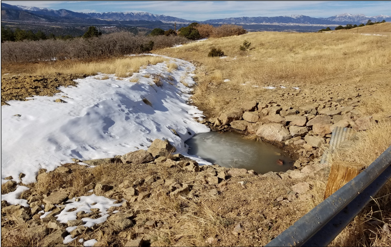
Photo 3. The disturbance at the culvert inlet has been seeded and hydro-mulched. Rock rip/rap and sediment trap has been installed. Lat/Long:37.69730,-105.19998
