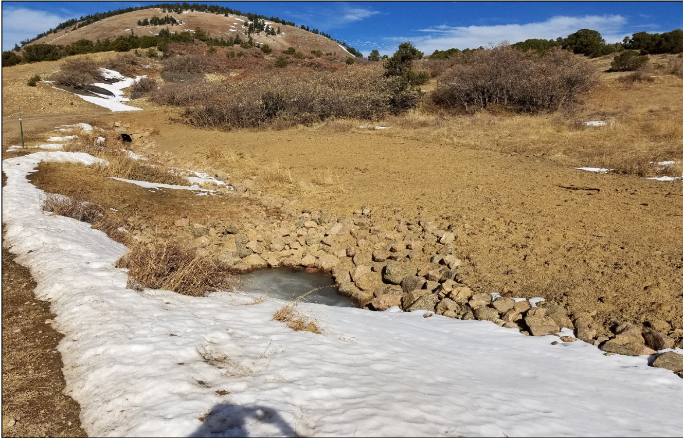
Photo 2. The disturbance at the culvert inlet has been seeded and hydro-mulched. Rock rip/rap has been installed. Lat/Long:37.69730,-105.19998
