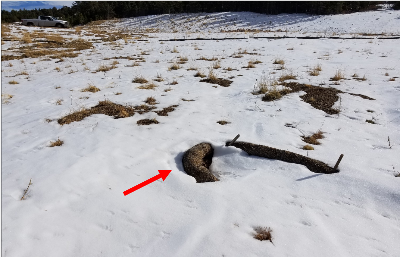
Photo 9. This photo shows the wattle displaced.
