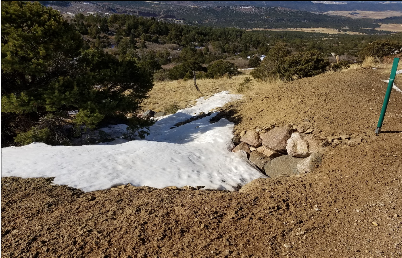
Photo 1. Outlet protection has been installed and disturbance area was hydro mulched. Lat/Long:37.69799,-105.20237.
