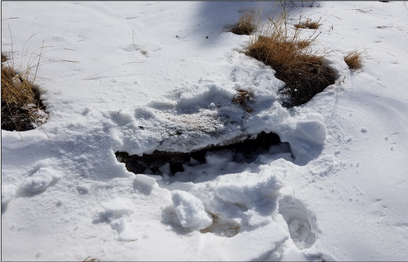
Photo 10. This wattle was filled in with sediment and erosion undercut.
