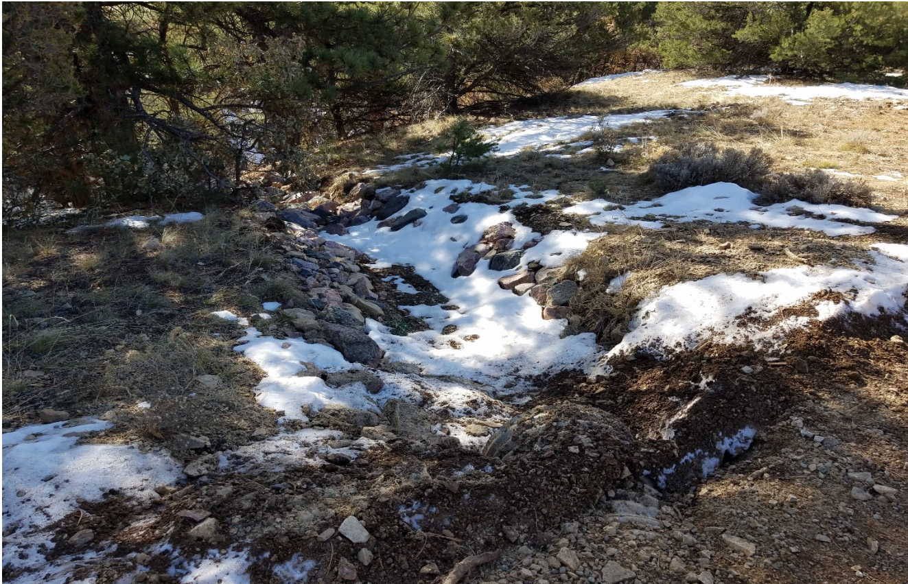
Photo 6. Erosion channel has been repaired at the culvert outlet. Rock rip/rap and erosion matting was placed in channel. Lat/Long:37.70004,-105.21143
