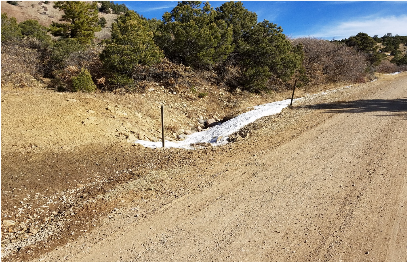
Photo 7. The disturbance along the side of the access road has been seeded and hydro-mulched. Inlet protection is installed at the culvert.
