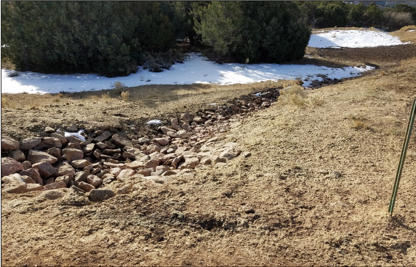
Photo 2. The culvert outlet protection has been installed.
