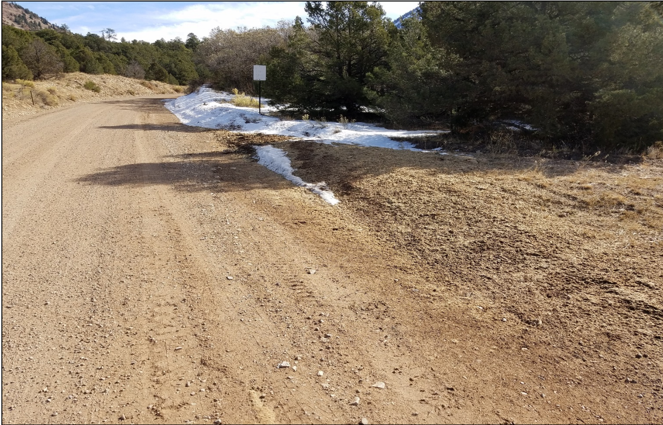
Photo 1. The disturbance along the side of the access road has been seeded and hydro-mulched.
