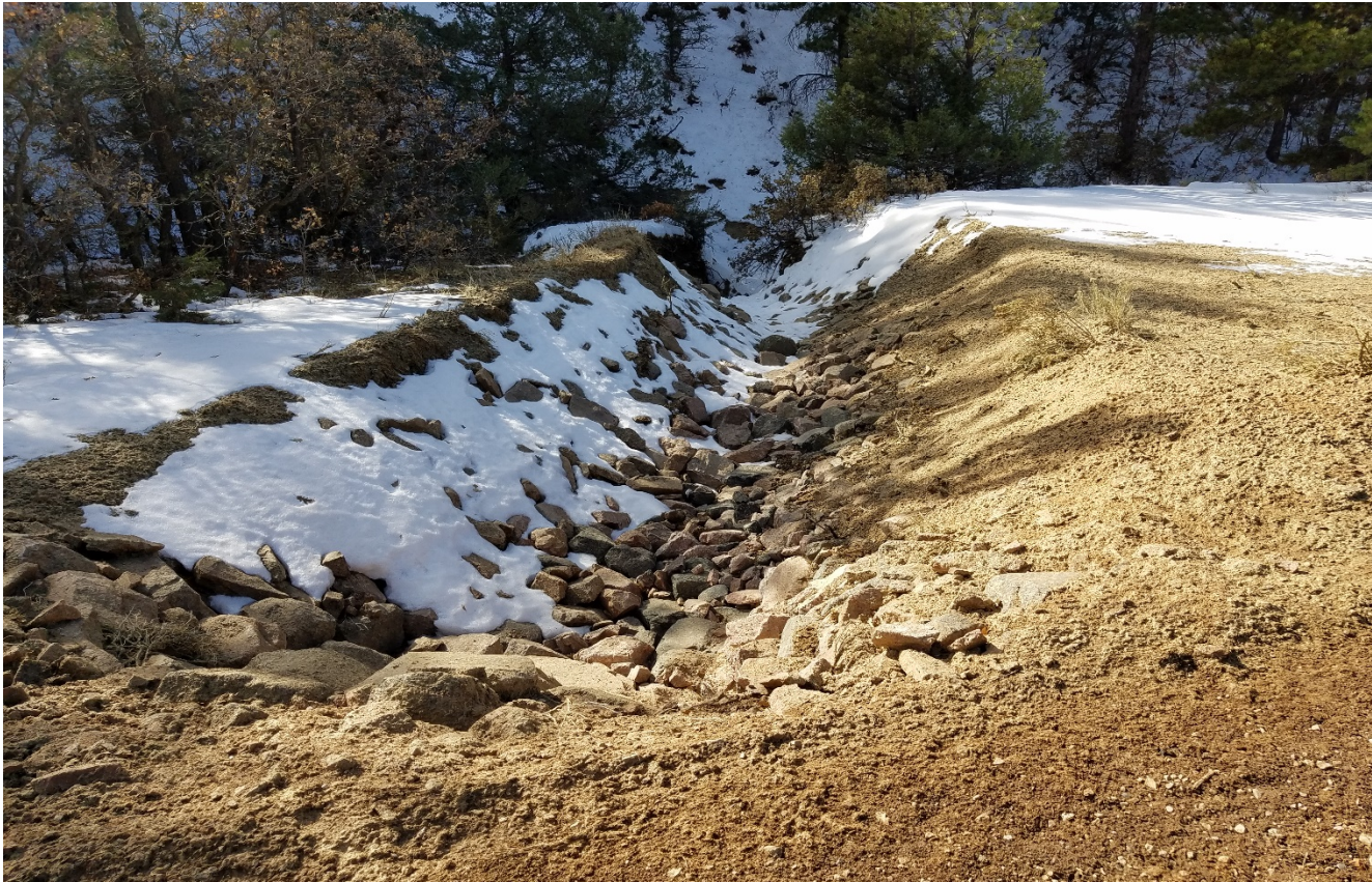
Photo 3. Erosion channel has been repaired at the culvert outlet. Rock rip/rap, wattles, and erosion matting was placed in channel. Larger rip rap was installed.
