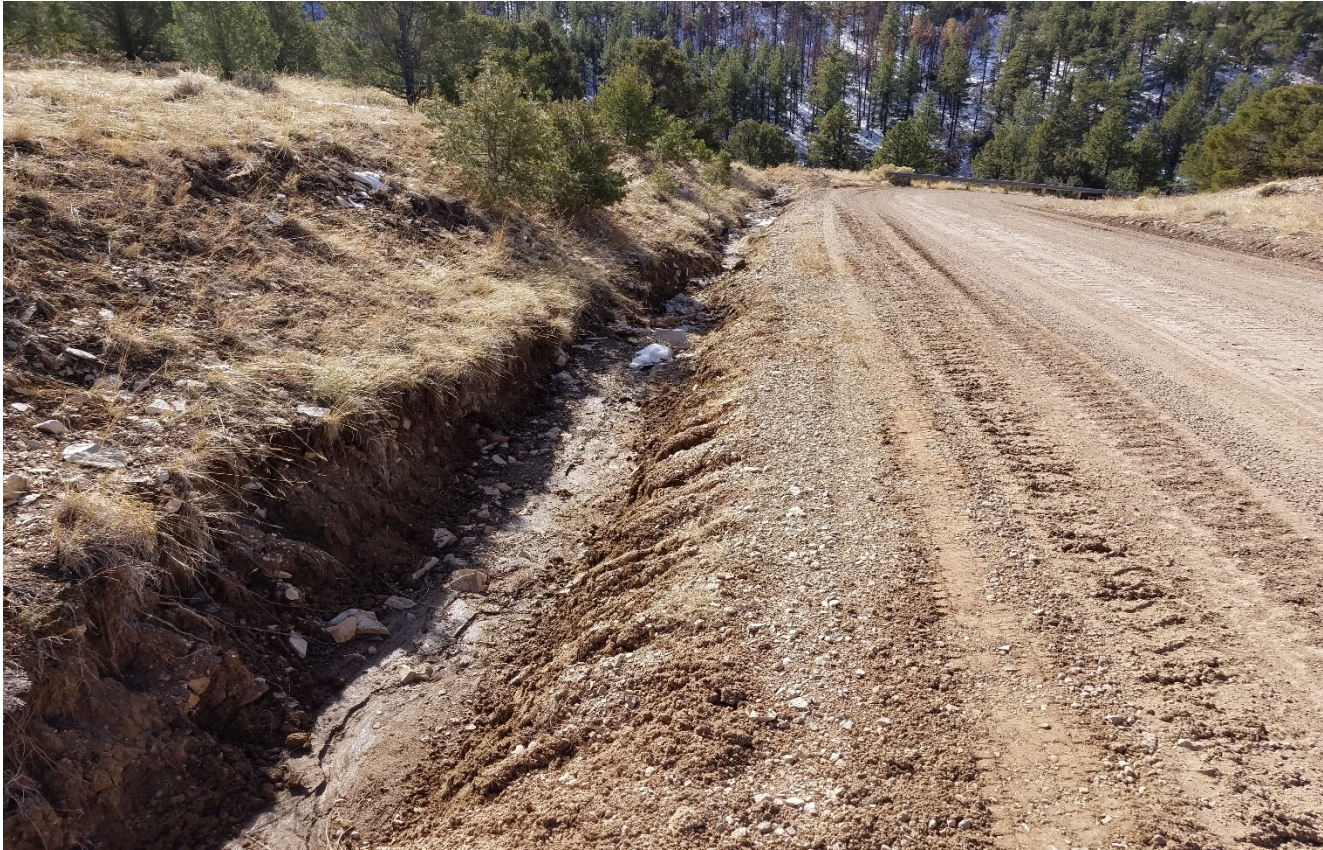
Photo 4. Facing south. This area along the side of the road has a deep erosion channel and BMP's have not been repaired. Lat/Long:37.69860,-105.21673
