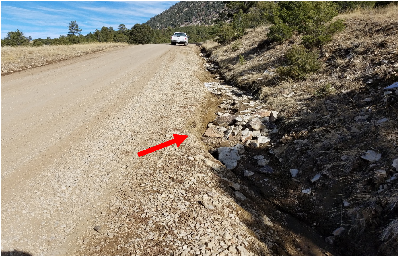
Photo 5. Facing north. This area along the side of the road has a deep erosion channel and BMP's have not been repaired. Rock check dams have been displaced. As stated in the previous inspection "Stormwater will flow toward the side and will erode the into road." Lat/Long:37.69860,-105.21673
