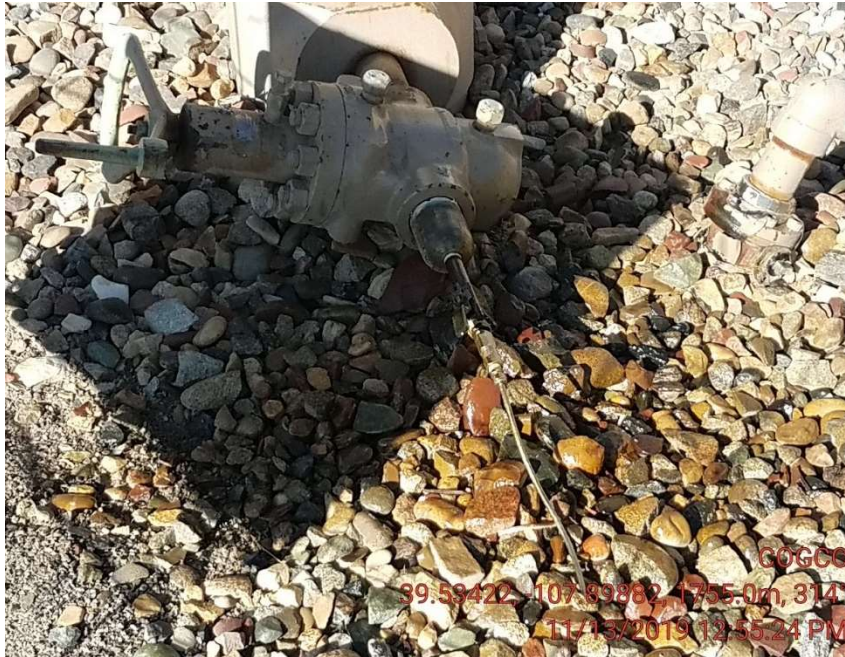
Valve leaking
