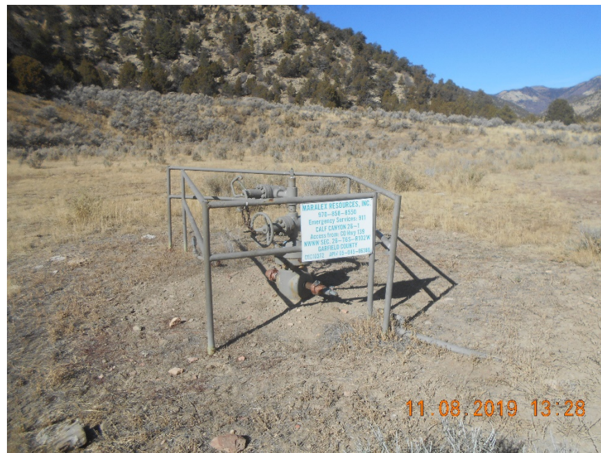
Wellhead with fence and sign. Temporarily abandoned with disconnected flowlines.
