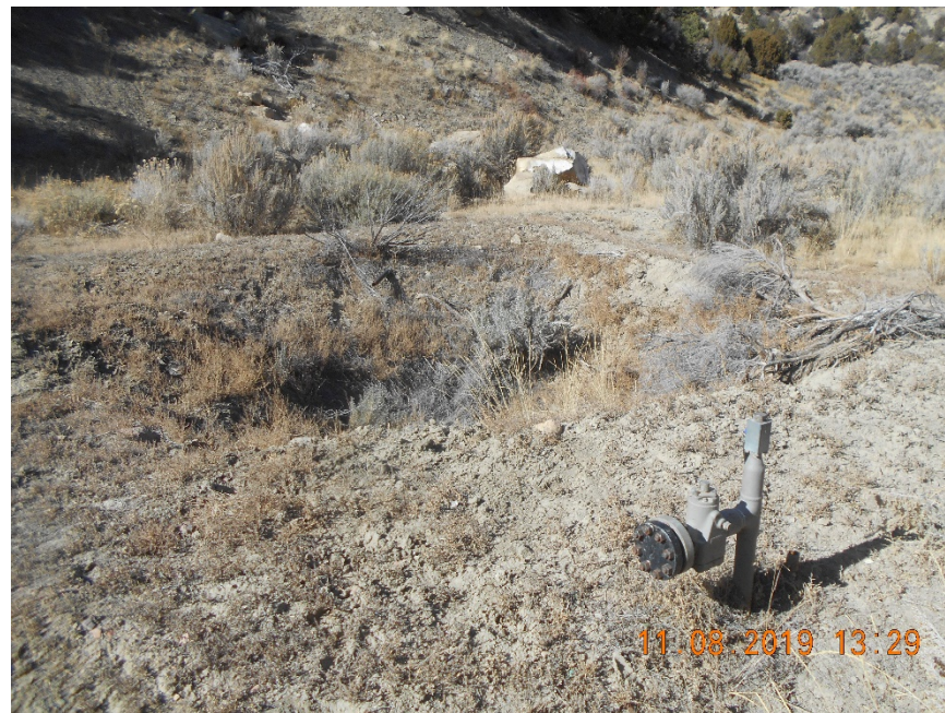
Flowline riser with blind flange. Blowdown pit.
