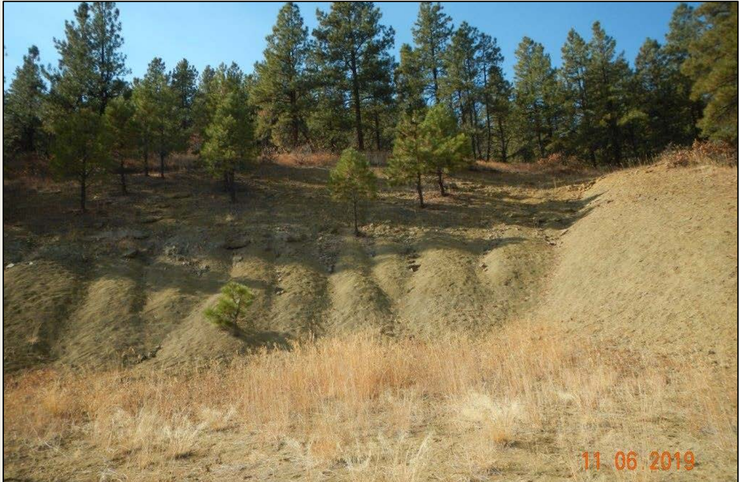
Photo 3. View of western cut-slope. Bare soils, erosional channeling and sedimentation observed.
