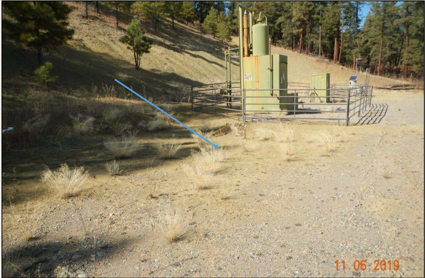
Photo 4. View of sediment deposition (blue arrow) that flows onto the well pad and around facilities.
