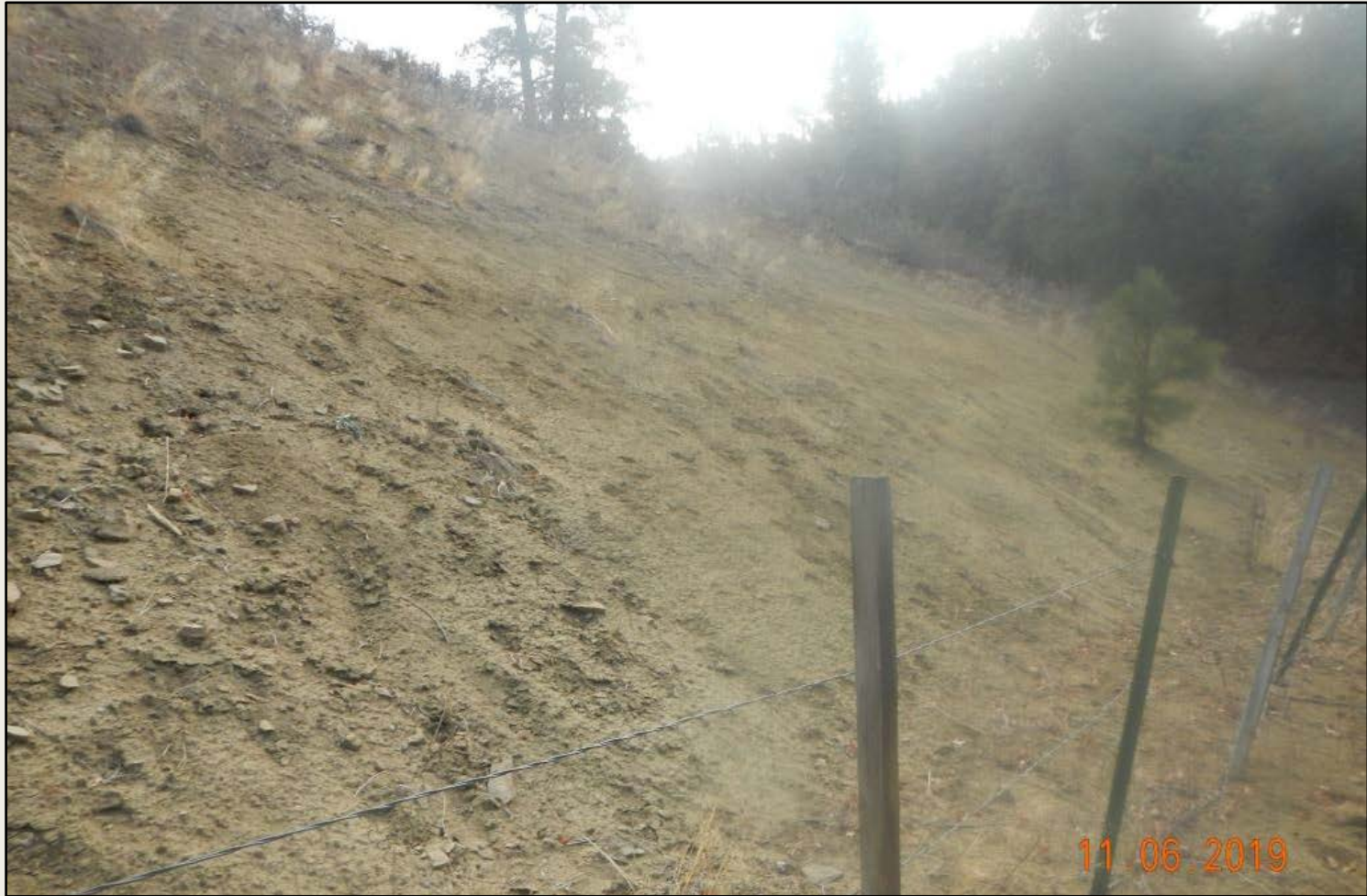
Photo 3. View of well pad cut-slope, largely with bare soils on lower slope and sparse grasses such as Indian ricegrass on upper portion of slope.
