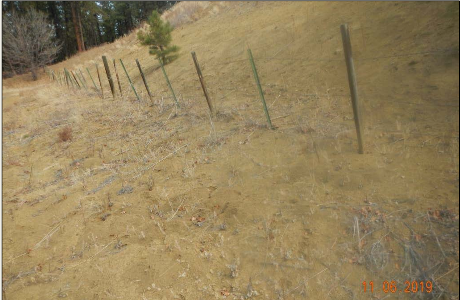
Photo 4. View of sediment deposition at the toe of the well pad cut slope.
