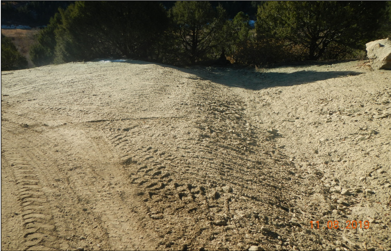
Photo 2. This drainage channel at the switchback of the road may require a sediment trap to slow the stormwater velocity to prevent erosion.
