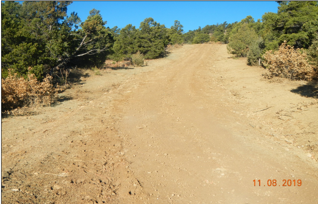
Photo 5. Facing west along the access road as it ascends the hill. Additional BMP's are needed to prevent erosion along the side of the road.
