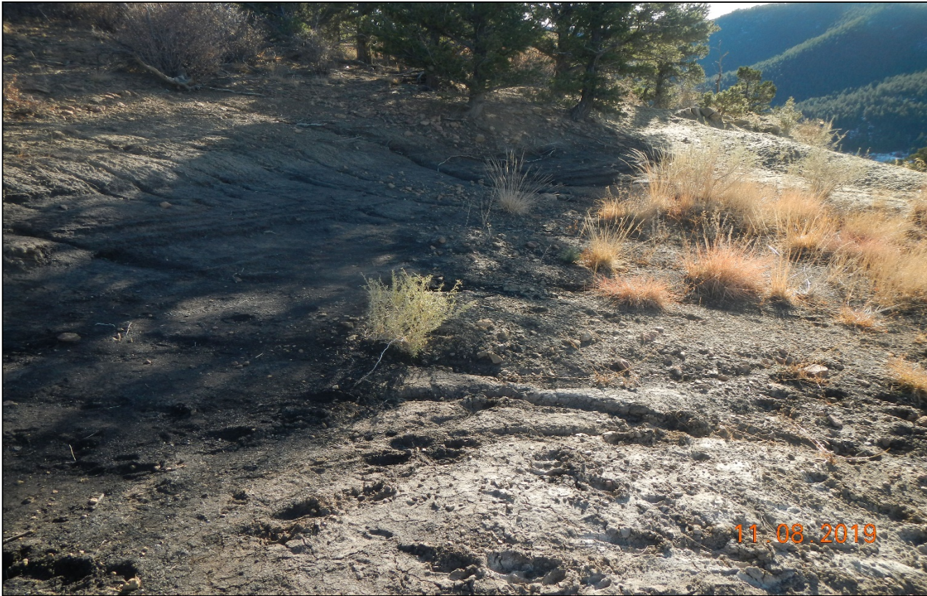
Photo 8. The east cut slope area is bare of vegetation and needs to be stabilized. Soil is needed in this area to establish vegetation.
