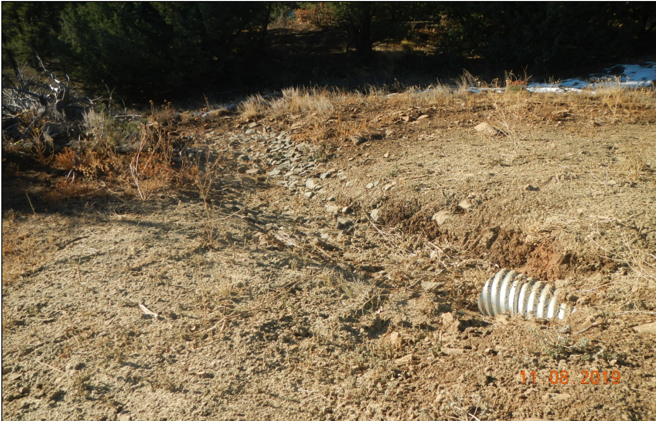
Photo 4. There is rock rip/rap in the culvert outlet but additional BMP's may be needed to slow the stormwater velocity.
