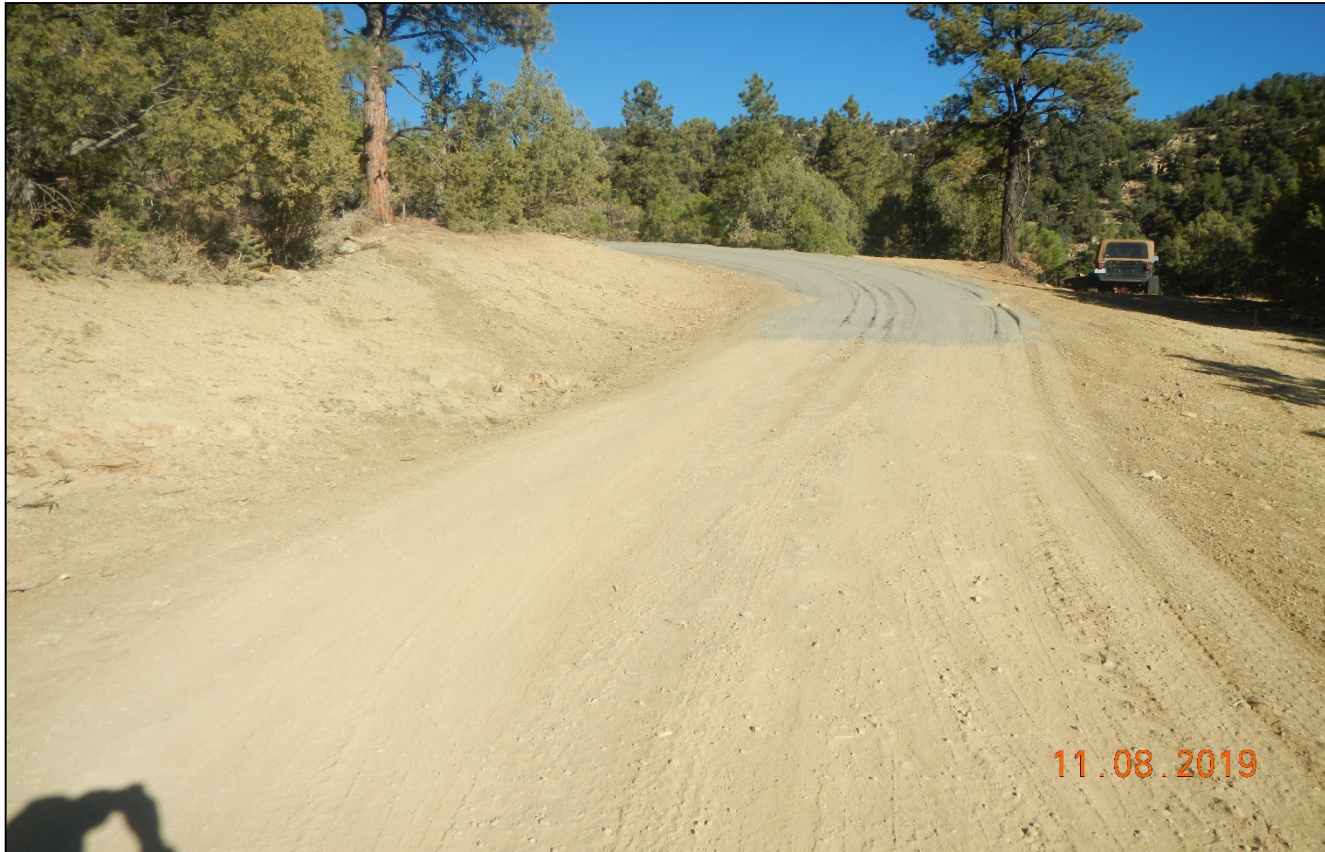
Photo 1. The access road has been regraded and gravel is being spread along the surface.
