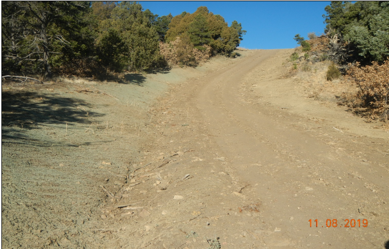
Photo 6. Facing west along the access road as it ascends the hill. Additional BMP's are needed to prevent erosion along the side of the road.
