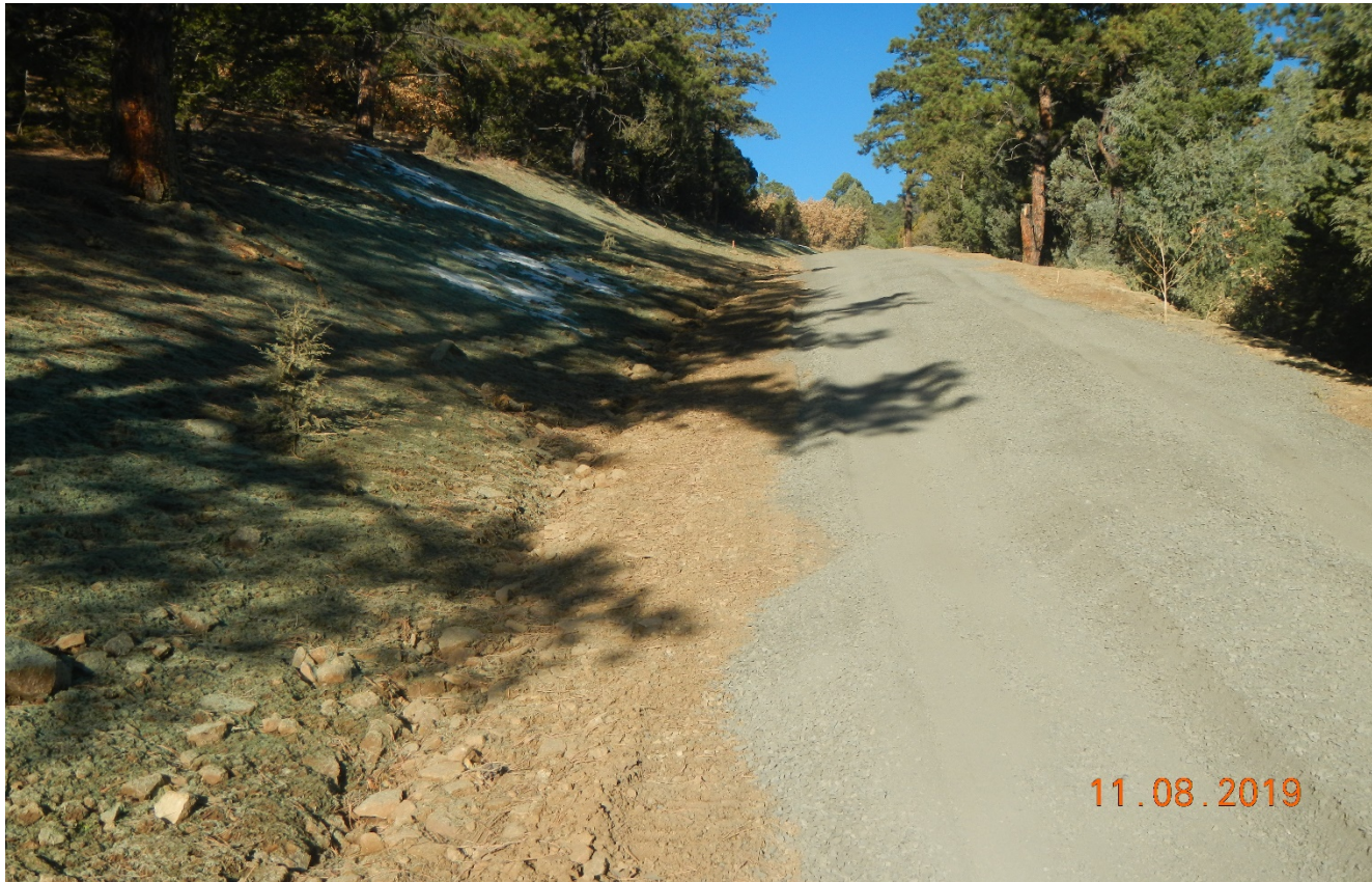
Photo 3. Facing west along the access road as it ascends the hill. The sides of the road are hydromulched.
