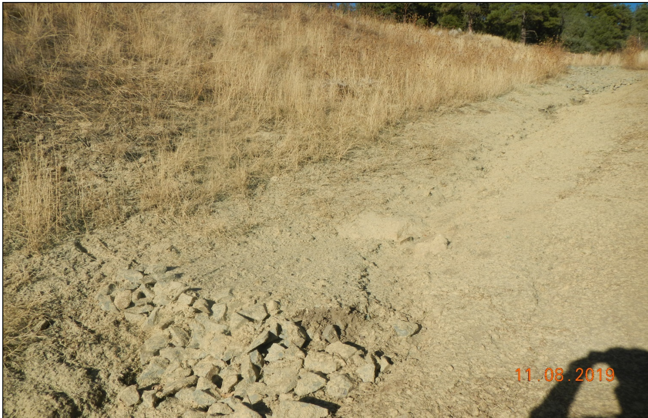
Photo 6. Sediment has filled into the check dam which requires maintenance.
