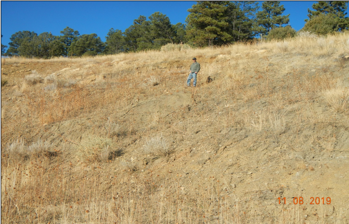
Photo 9. There is a soil slough where I am standing in the photo along the cut slope. There is erosion along the cut slope which is not stabilized.
