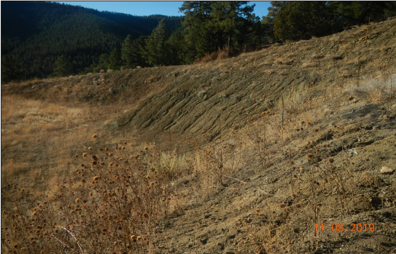
Photo 10. Facing southwest along the cut slope, There is erosion along the cut slope which is unstable.
