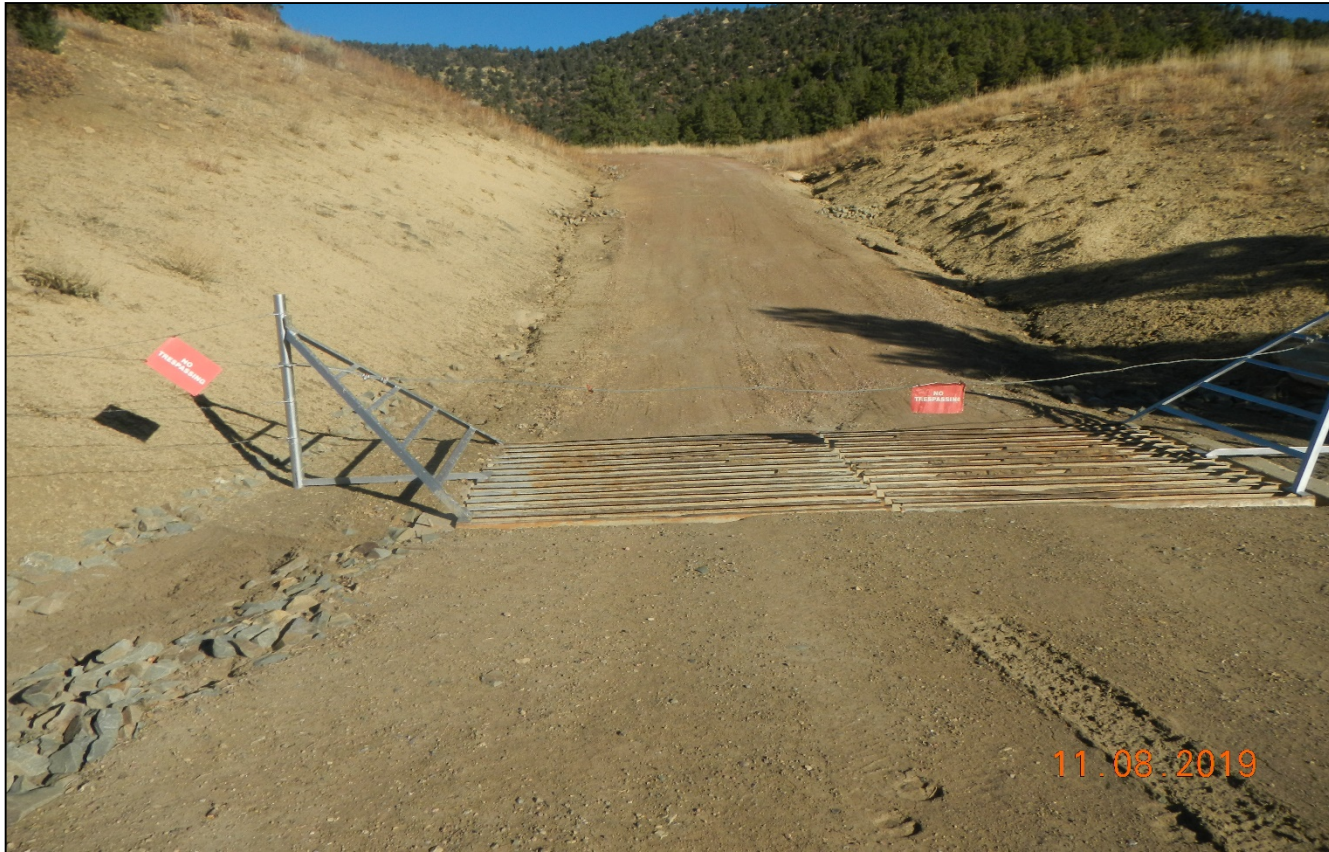
Photo 1. Facing north at the beginning of the access road. The cattle guard has been maintained and slopes have been hydro-mulched.
