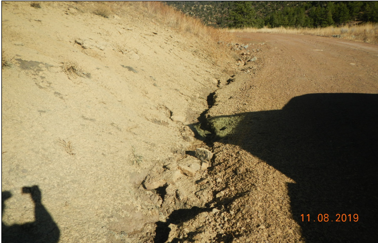
Photo 4. Erosion channel is developing along the side of the road which need to be repaired and controlled.
