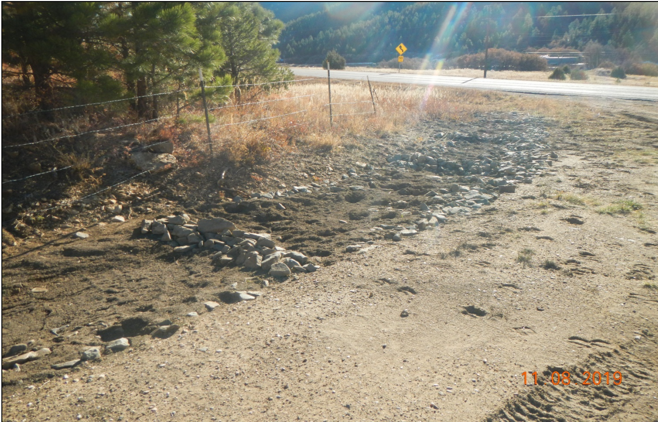
Photo 2. Rock rip/rap was installed on the side of the road at the beginning of the access road. Sediment has filled into rip rap indicating erosion is not controlled.
