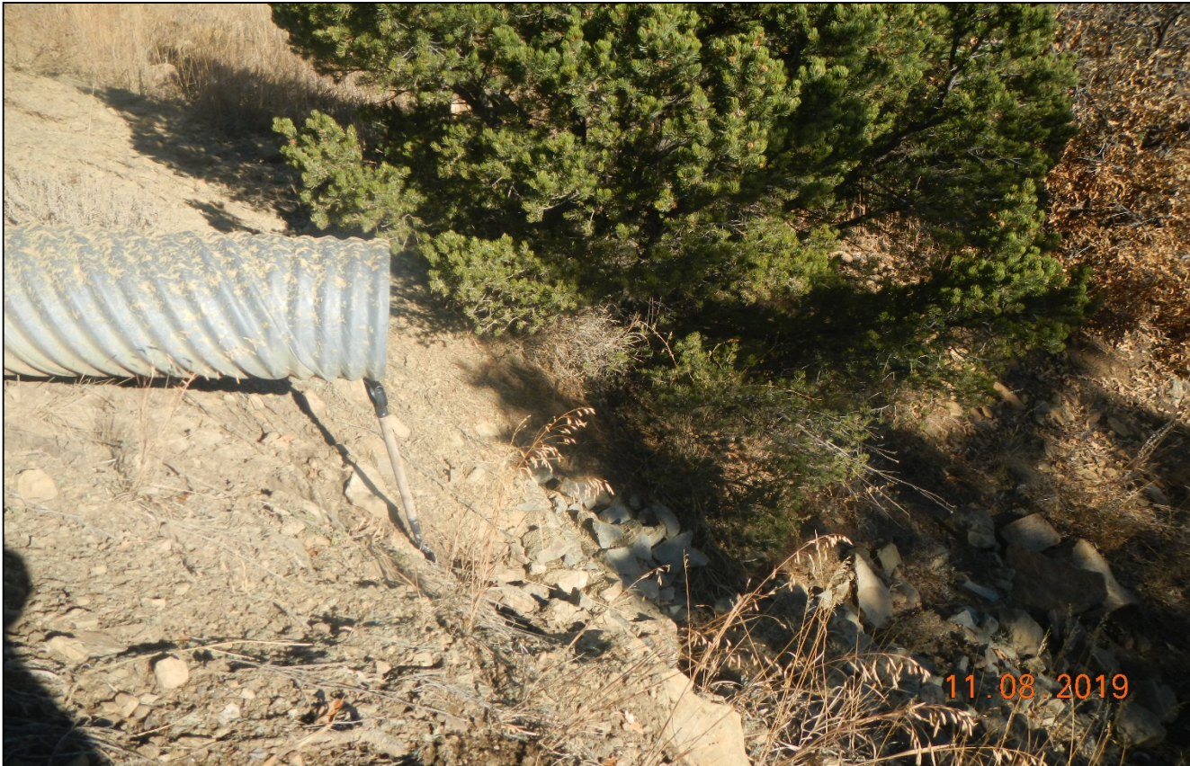
Photo 5. The culvert outlet extends to far out from the road which creates a 3 ft. vertical drop for stormwater which can accelerate erosion. The outlet protection is not adequate and the culvert should be cut closer to the road.
