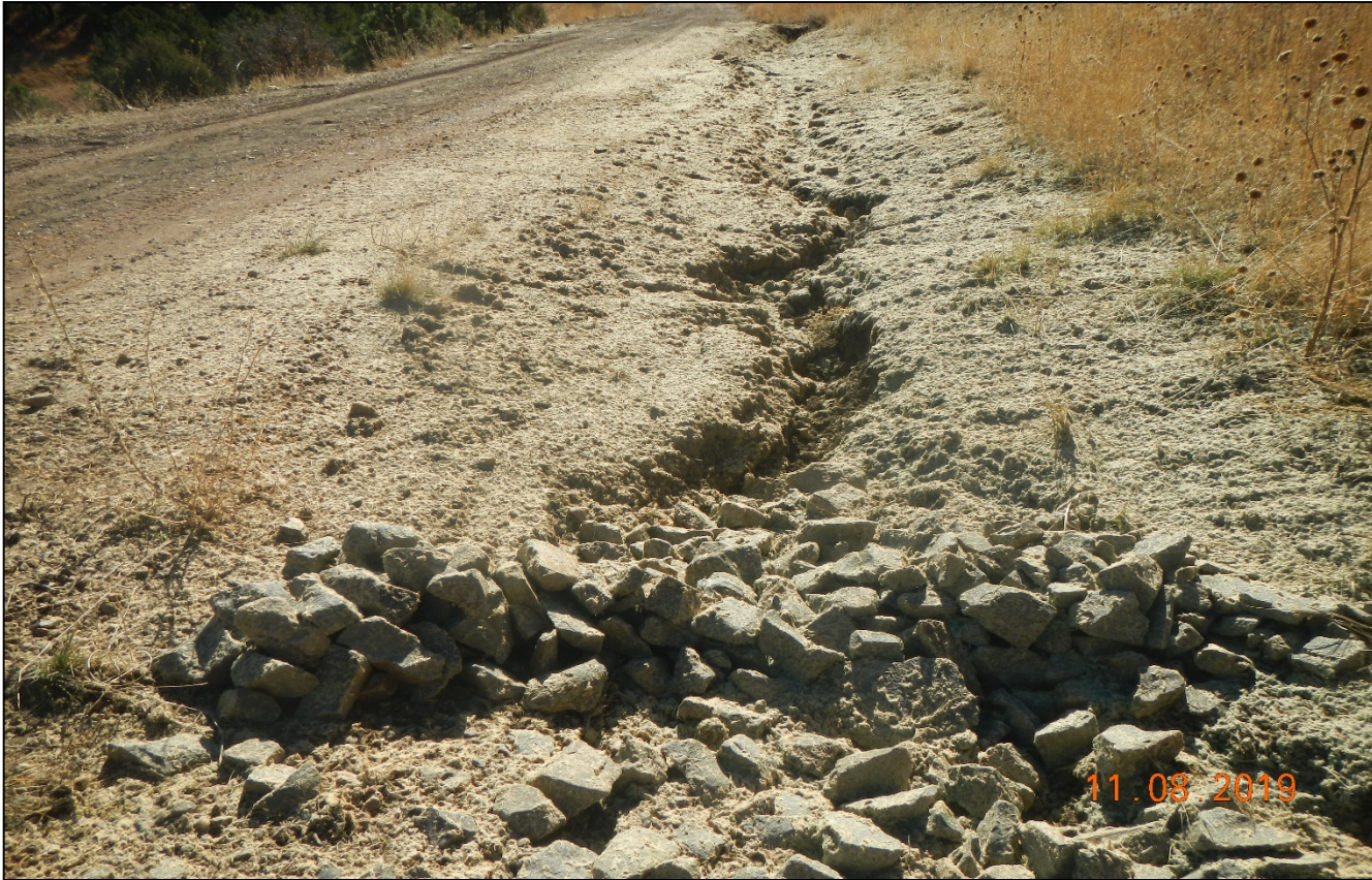
Photo 7. There is an erosion channel developing beyond the check dam which needs to be repaired.
