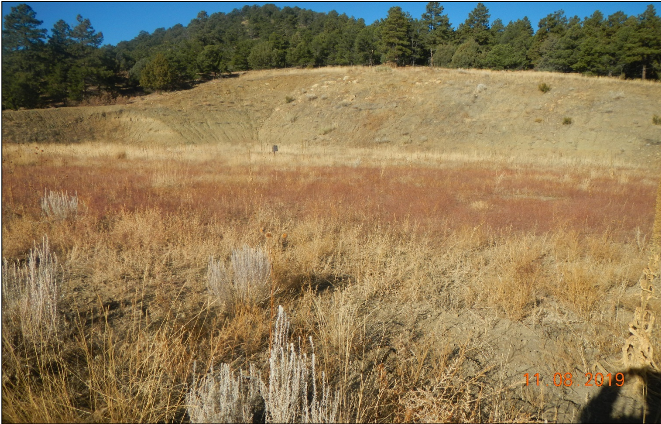
Photo 12. Facing northwest toward the location. The cut slope is bare of vegetation and not stabilized.
