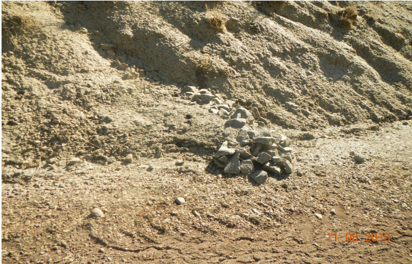
Photo 3. Rock check dams were installed along the road however, sediment has filled in the check dams. The check dams were not properly installed by trenching the sides into ground and creating a low area in the center of the check dams.
