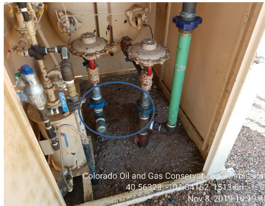
Photo 14: Stained soil in west separator house (facing tank battery)
