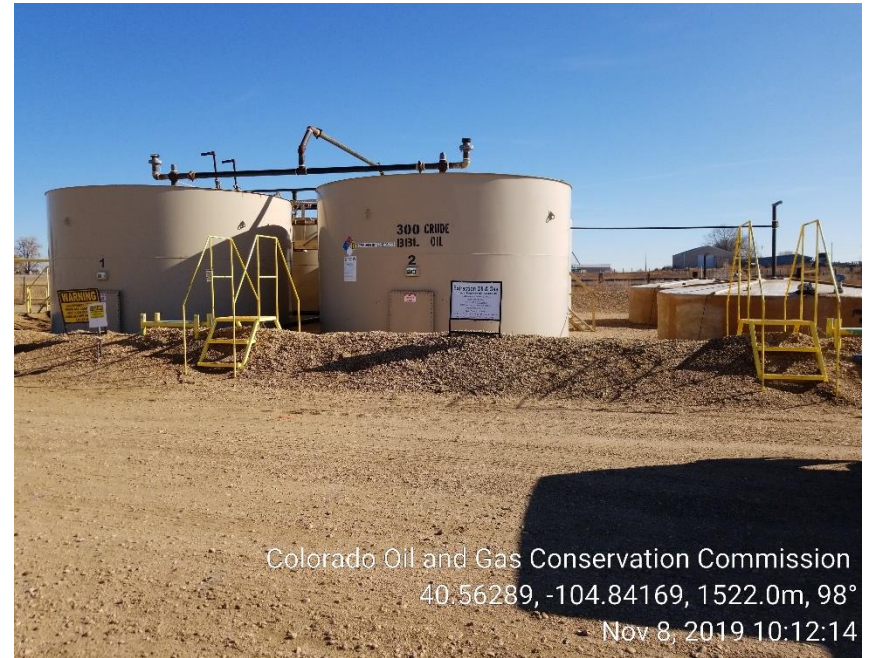
Photo 2: Tank Battery
