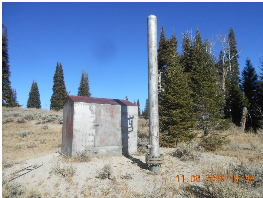
Meter housing and dehydrator. Disconnected.
