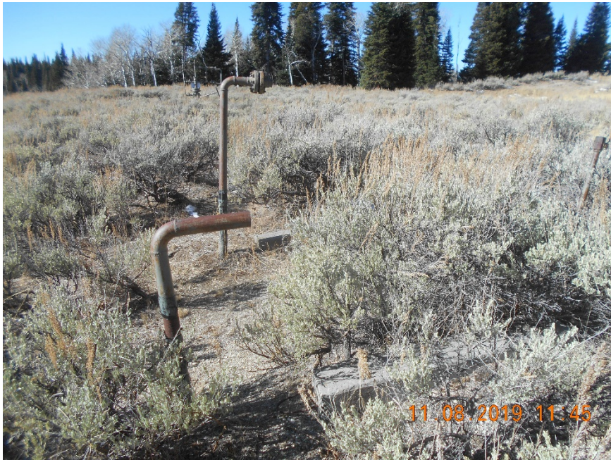
Multiple flowline risers. 2x2" & 1x1" disconnected. Not locked out/tagged out or marked.
