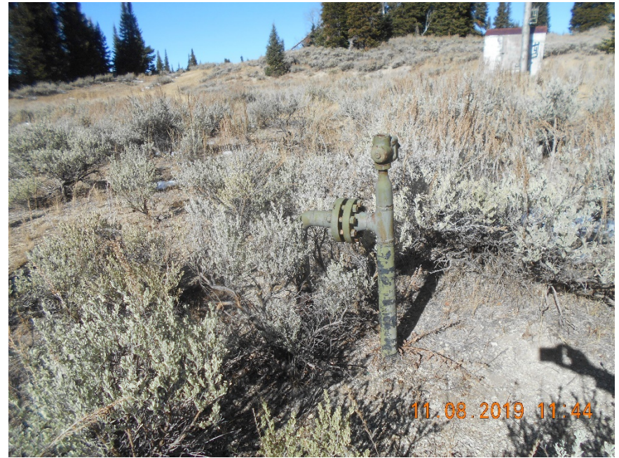
Flowline riser. 2x2" disconnected. Not locked out/tagged out or marked.
