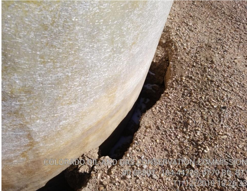
Pic 5 water tank no labels/erosion issues
