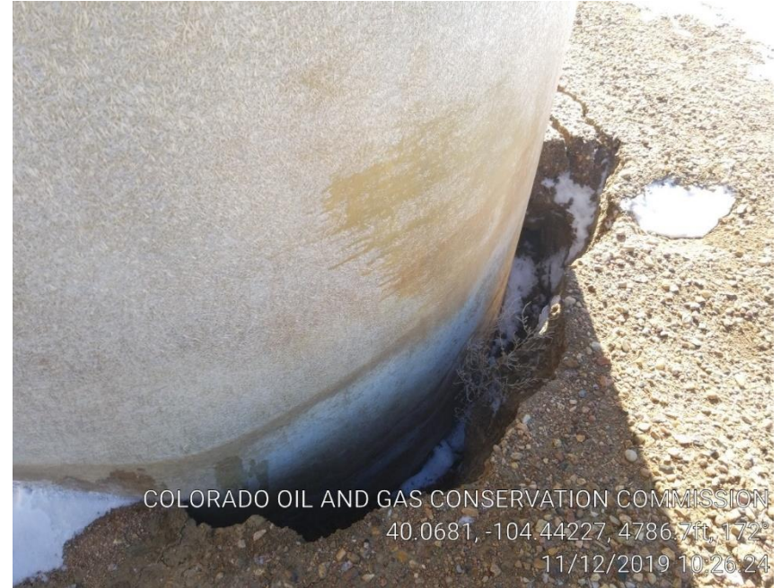
Pic 4 water tank no labels, erosion issues
