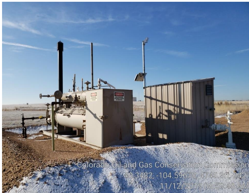
Photo #3 Separator & Meter Run
