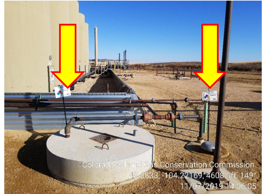
Photo 4 – East Tank Battery SW corner. Capacity is missing from signs.
