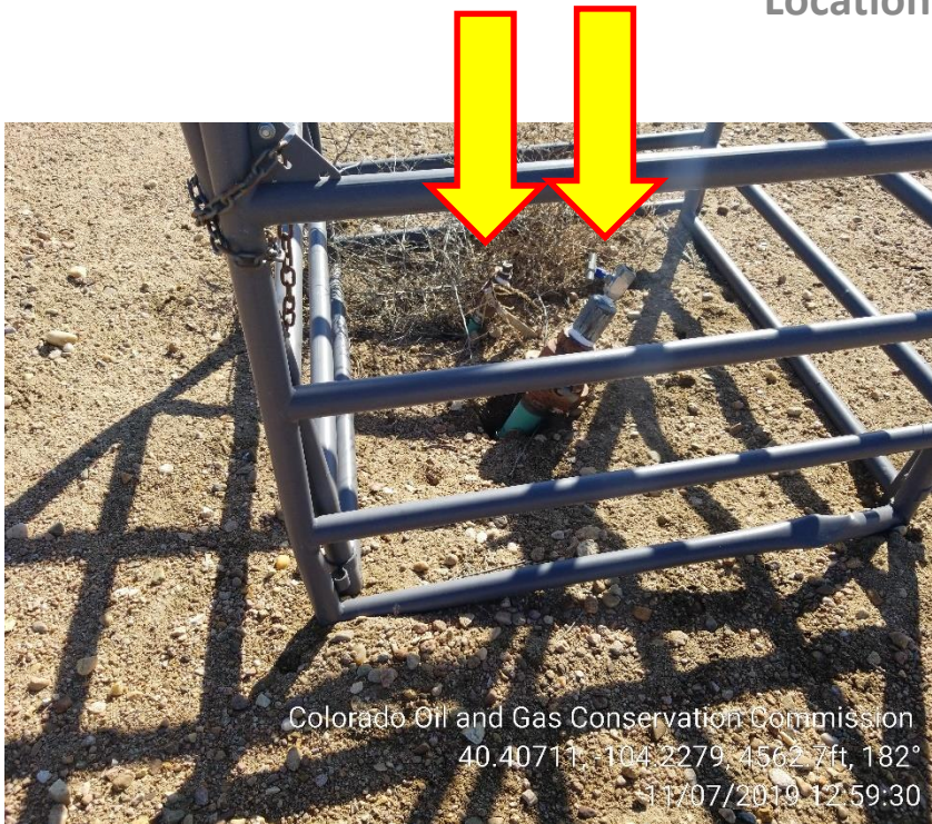
Photo 3 – Unmarked 1" and 2" Risers, West of Separator
