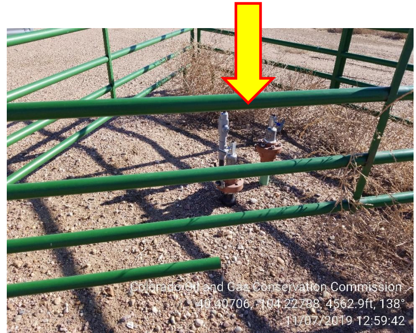
Photo 4 – Unmarked 1" and 2" Risers, West of Separator
