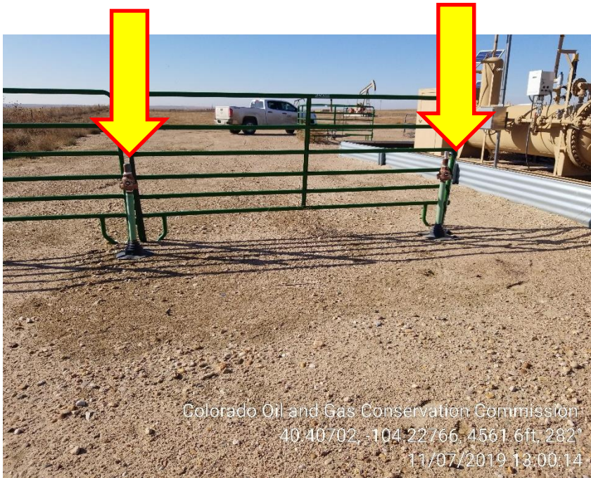
Photo 5 – Unmarked 1" and 2" Risers, South of Separator
