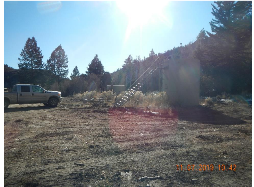
Equipment removal in process
