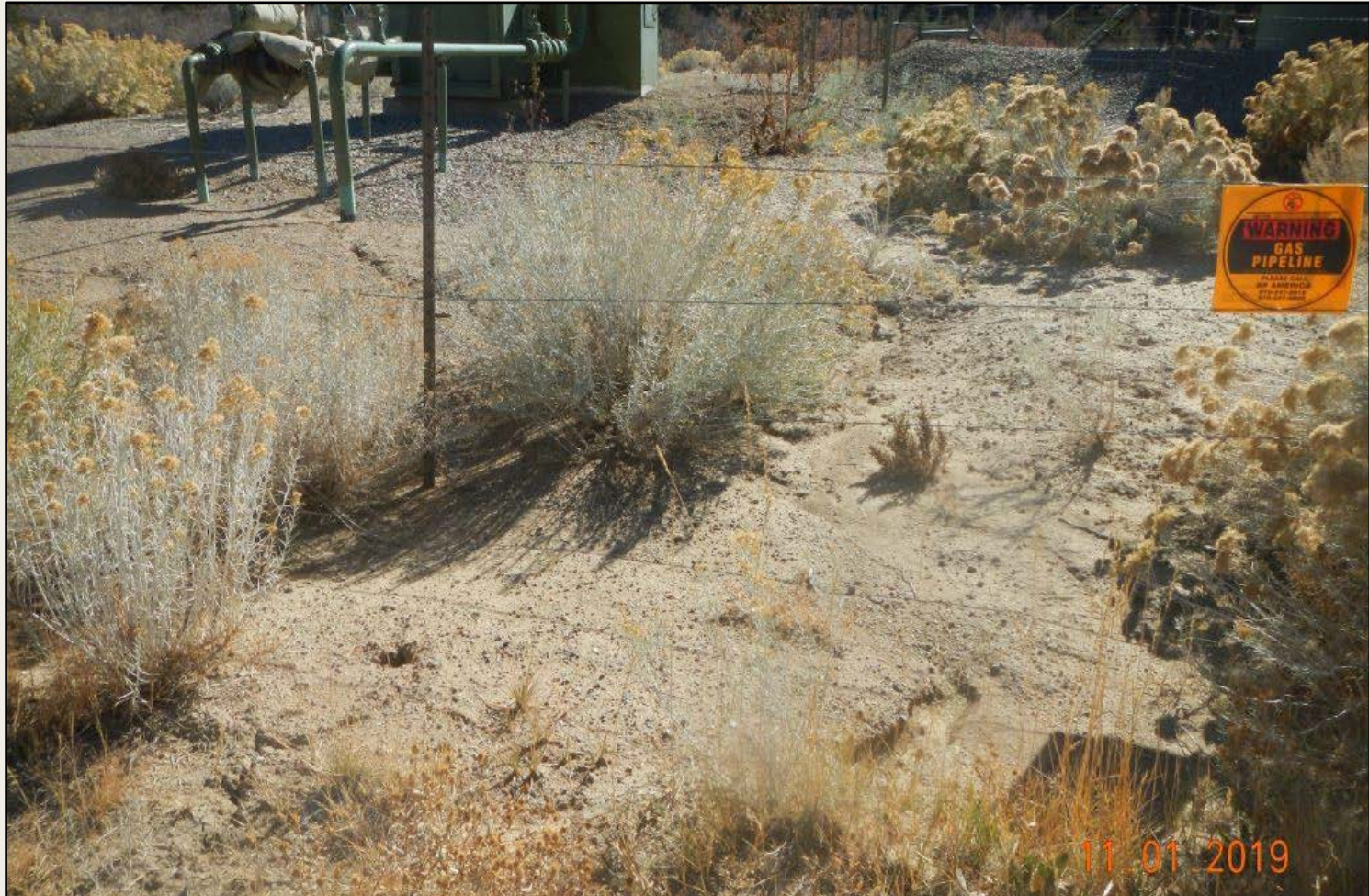
Photo 3. View of area adjacent to the northern facilities where stormwater flows off of the well pad westward, and resulting in erosion within the northwestern project area.
