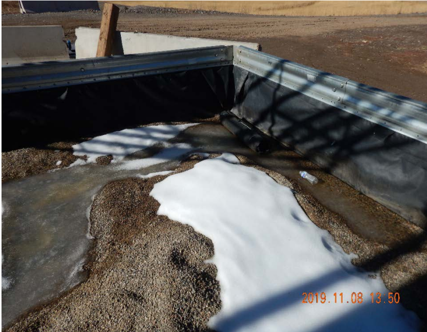
Photo #3 – Lined tank battery area contained snow/ice and fluids on inspection date. No hydrocarbon odors or sheen were observed during inspection. Note trash (water bottle) depicted inside northwest corner of tank battery.
