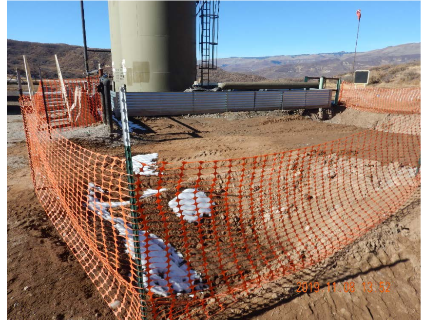
Photo #6 – View of fenced, scraped area east of tank battery from southeast corner. Open excavations were observed in southeast and northwest corners of this area on inspection date.
