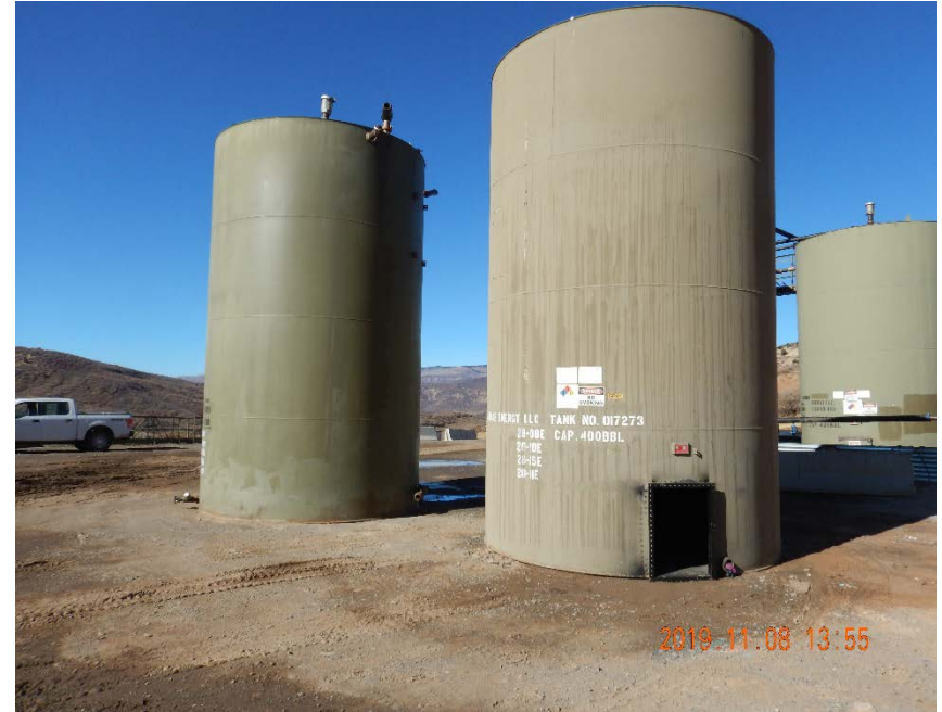
Photo #8 – View of unused 400 bbl ASTs from southeast. Note open access panel on east tank.
