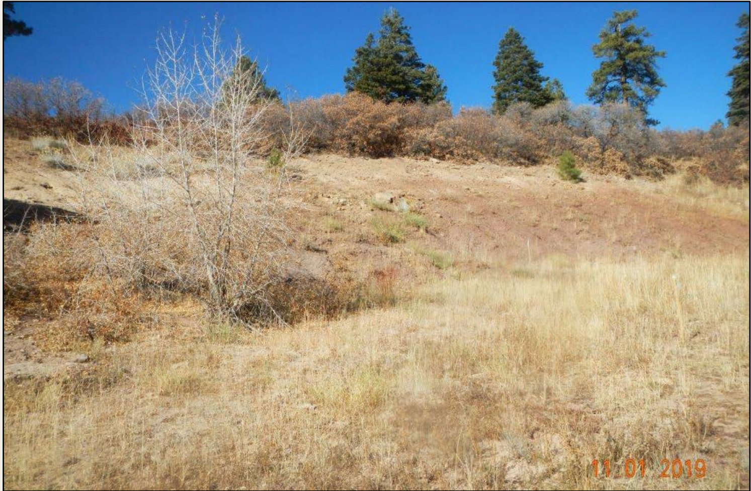
Photo 5. View of well pad cut-slope with poor revegetation. Rilling and scouring observed on bare soils.
