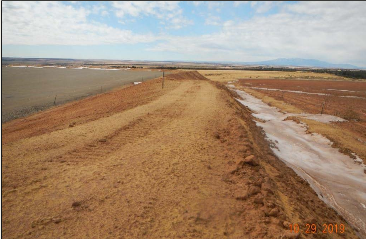
Photo 2. View of the northern fill slope from the northeastern corner facing westward. Disturbed soils are tracked and hydromulched. Drainage swales and berms are placed around the well pad perimeter.
