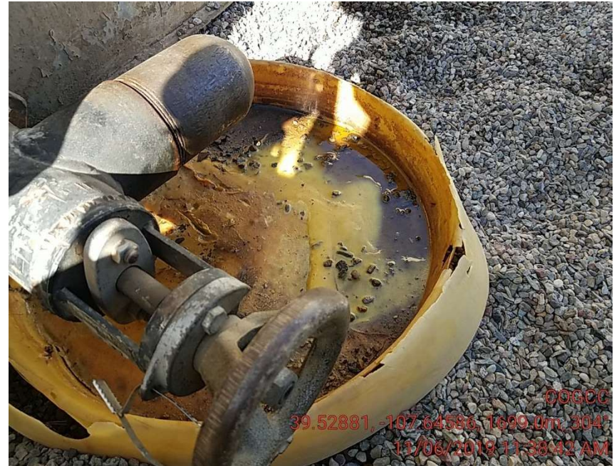
Condensate in drip pan next to tank burner that is running
