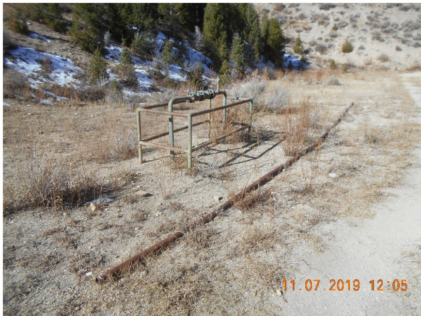
Flowline riser with junk 2" pipe.
