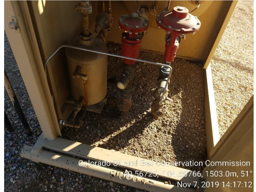
Photo 4: Stained soil removed from separator house
