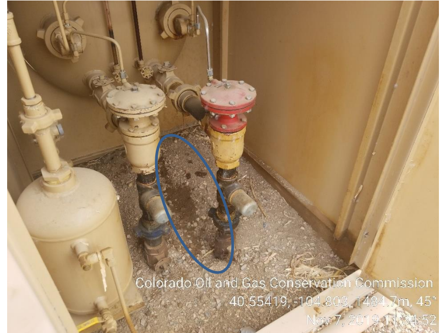
Photo 8: Stained soil in separator house.
