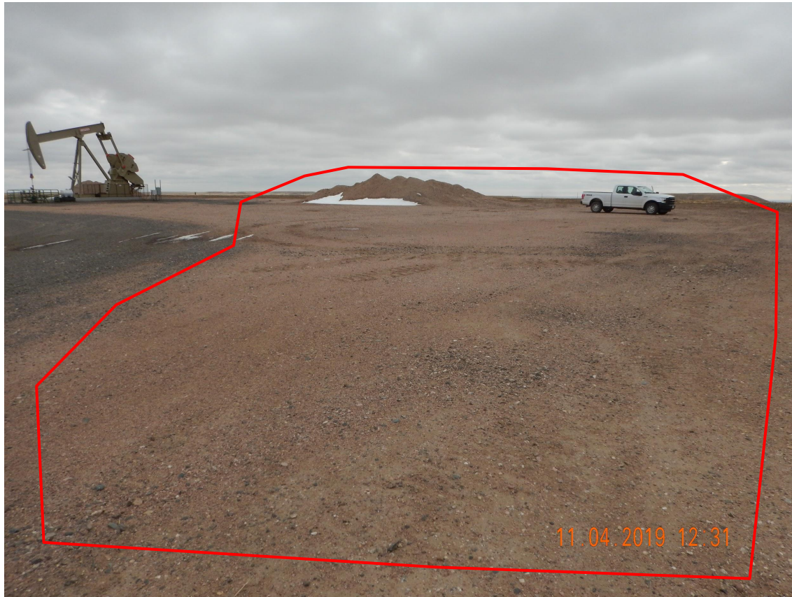
Photo 3. Photo taken from the western well pad, facing South. Photo illustrates that portions of the western and southwestern well pad can be further reduced in size to comply with Rule 1003. Currently, the Operator is storing gravel along a portion of this area where interim reclamation shall be performed.
