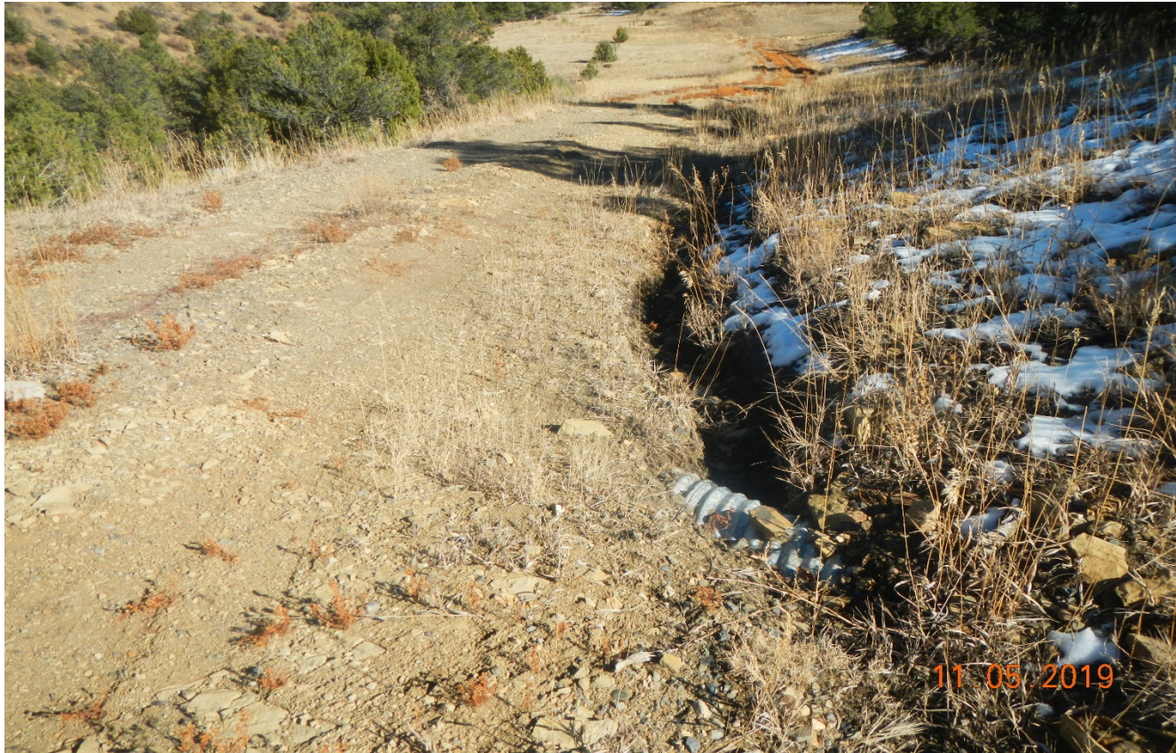
Photo 5. There is a culvert filled in with sediment.
