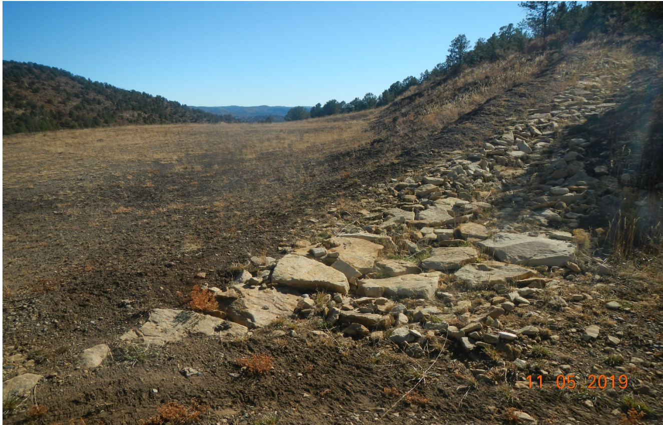
Photo 6. Facing southeast toward the location. There is a diversion ditch along the top of the cut slope with rock rip/rap installed.
