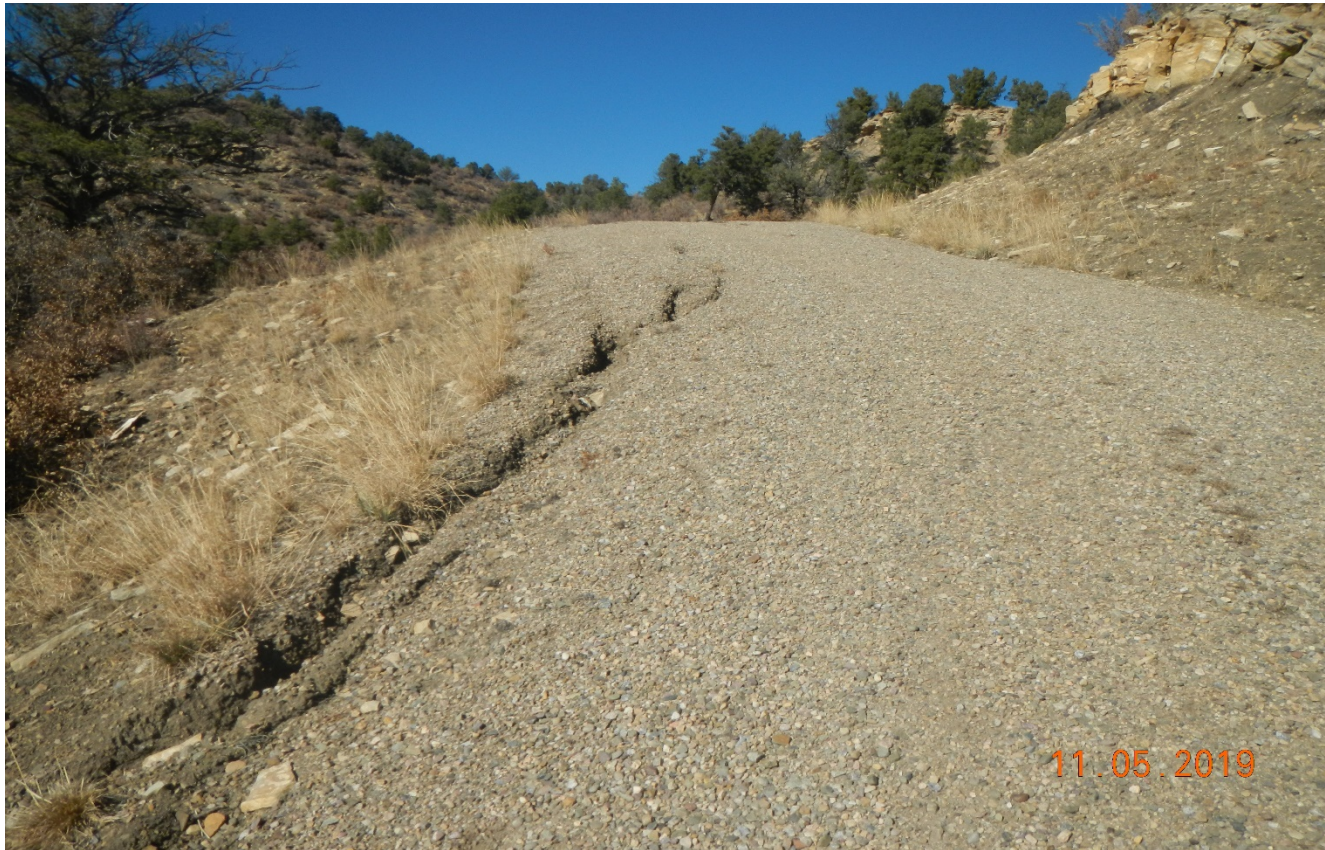
Photo 2. There is an area of erosion along the access road.
