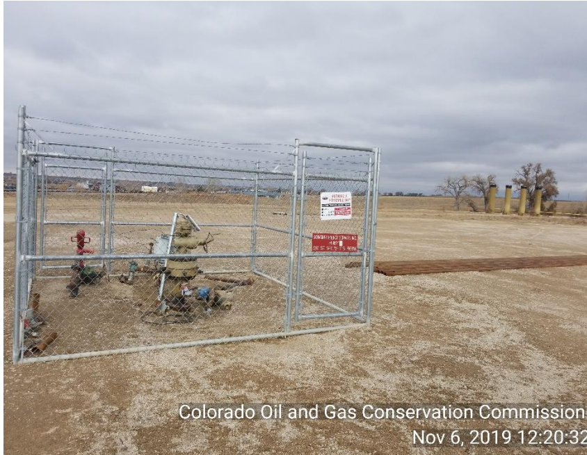
Photo 1 WH. All production equipment and flow lines have been removed from well head. Unused equipment: well head parts and tubing on location.
