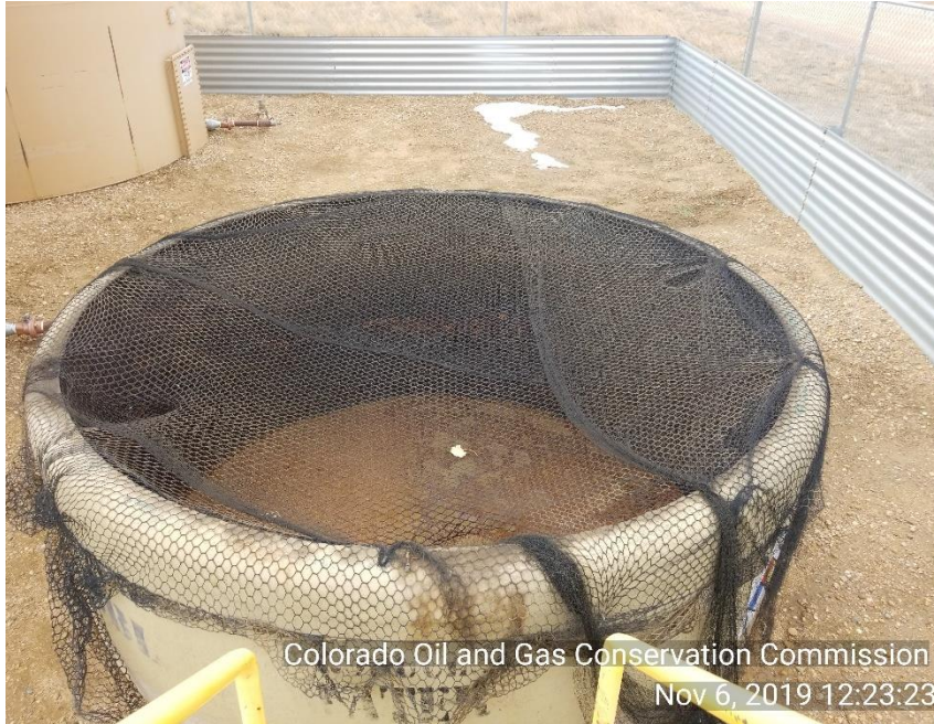
Photo 3 it appears bird netting has been repaired on produced water tank
