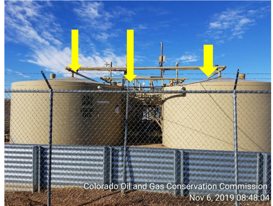
Photo 4 Flood plane anchor on crude oil tanks
