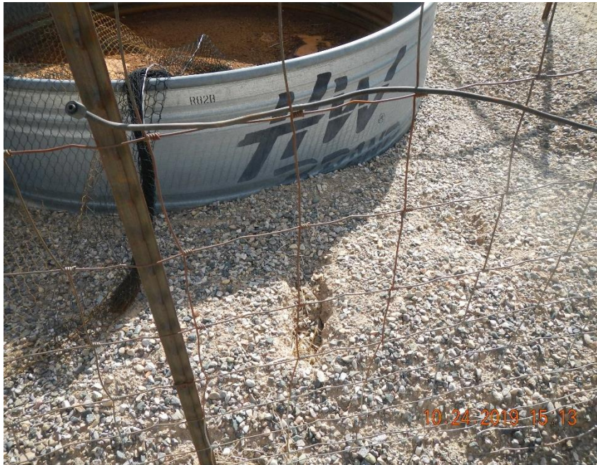
Secondary containment for produced water vessel has animal burrows in it and appears to be insufficient capacity.
