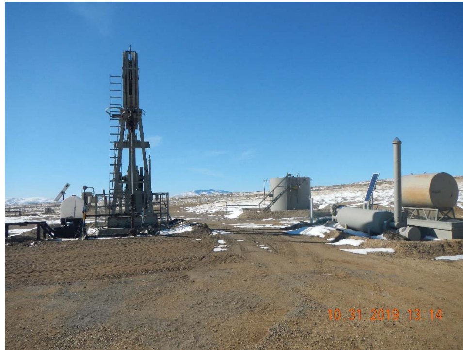
Photo 1. Overview of location taken facing west. Heated separator approximately 15 feet from wellhead.
