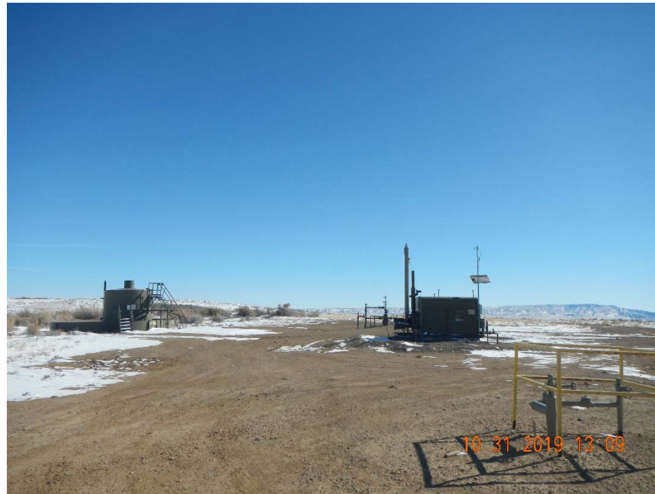
Photo 1. Overview of location taken facing southeast.
