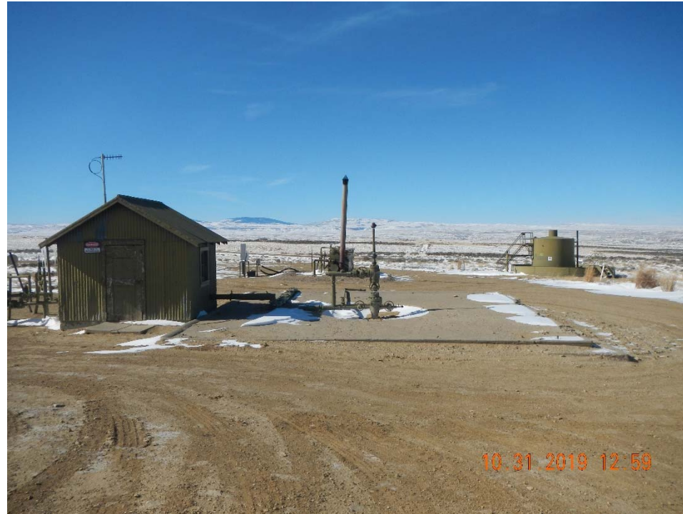
Photo 1. Overview of location taken facing northwest.
